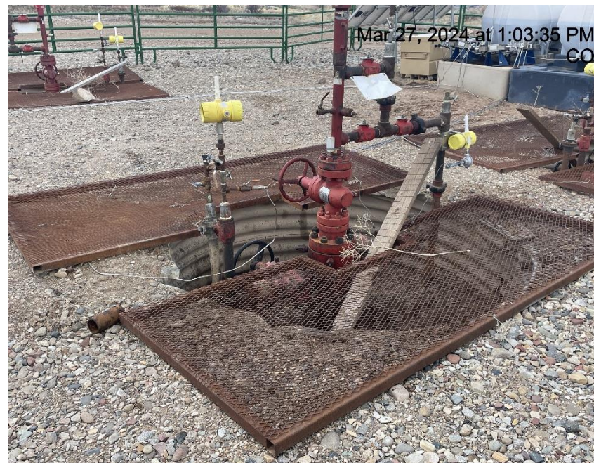
Photo # 1651 Cellar not properly covered/wildlife & personnel hazard
