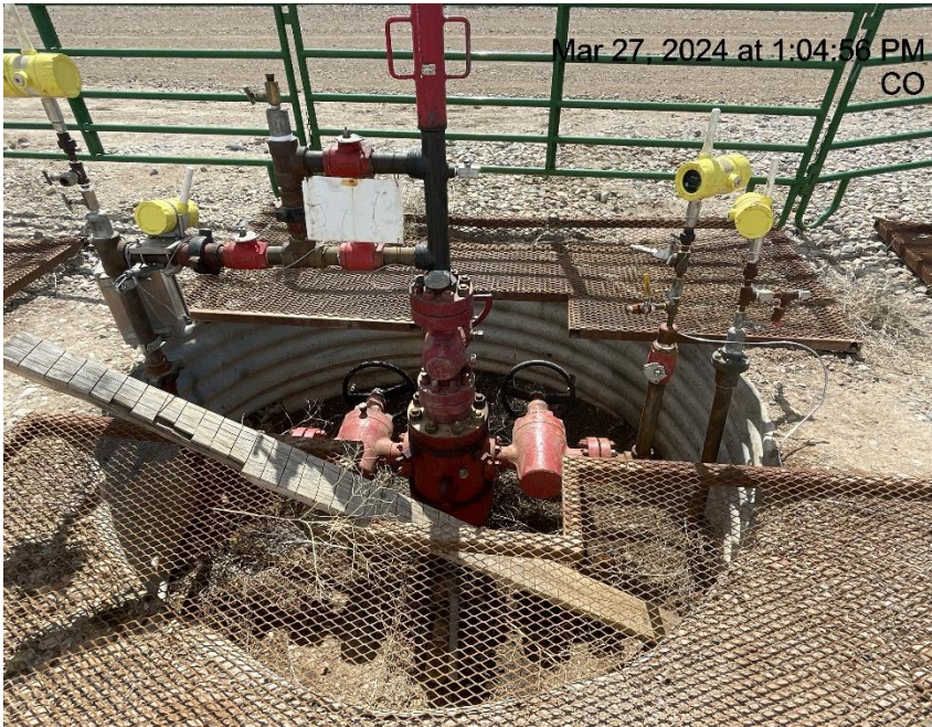
Photo # 1652 Cellar not properly covered/wildlife & personnel hazard
