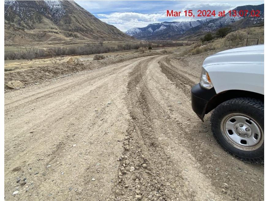
Insufficient Vehicle Tracking BMPs at Location Entrance/Exit – Photo #09938
