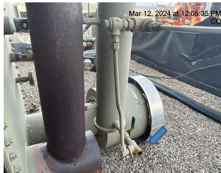
Photo # 9510 PRV vent line on tank burner terminates in an unsafe manner/does not comply with CECMC pressure safety device rules & general safety rules.
