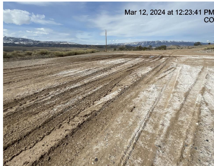
Photo # 9429 Lack of stabilization/compaction/insufficient tracking BMP's
