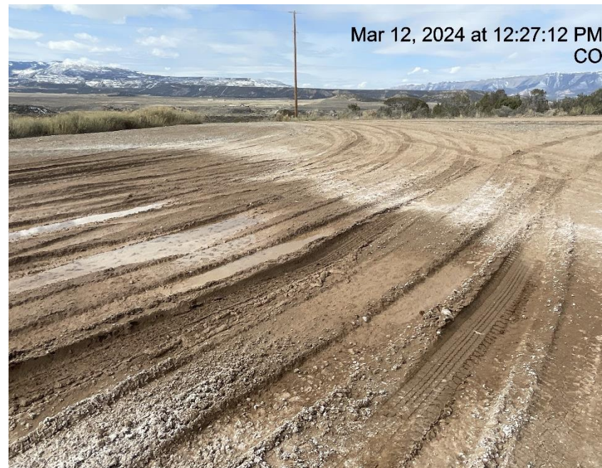
Photo # 9421 Lack of stabilization/compaction/insufficient tracking BMP's
