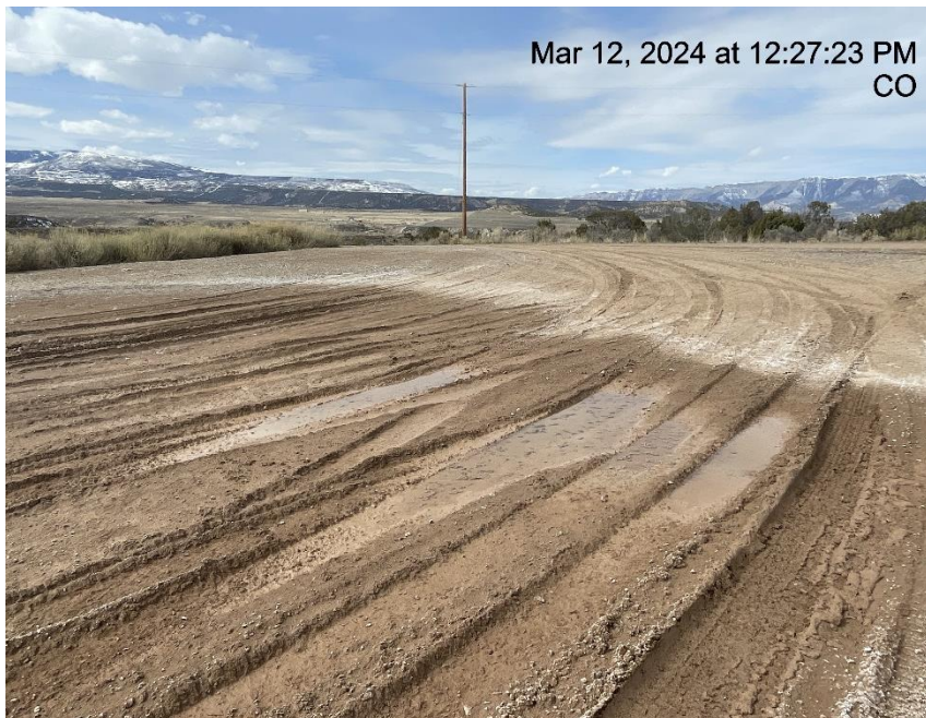
Photo # 9420 Lack of stabilization/compaction/insufficient tracking BMP's
