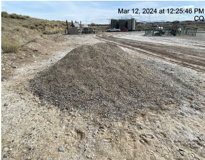
Photo # 9416 Stockpiled soils with no BMP's
