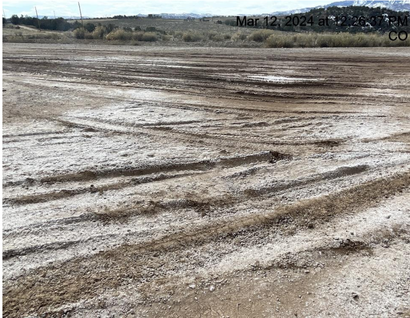
Photo # 9422 Lack of stabilization/compaction/insufficient tracking BMP's
