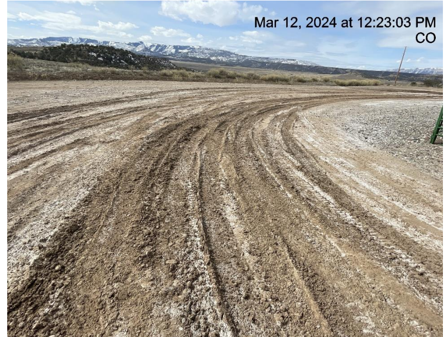
Photo # 9427 Lack of stabilization/compaction/insufficient tracking BMP's
