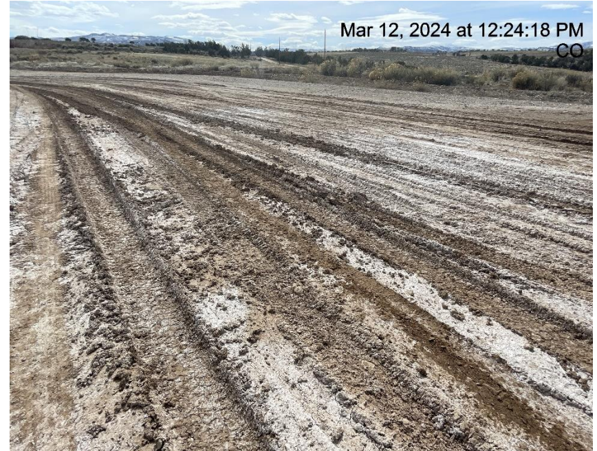
Photo # 9425 Lack of stabilization/compaction/insufficient tracking BMP's
