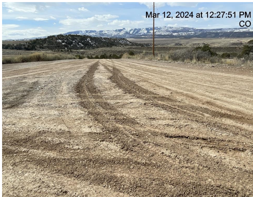
Photo # 9418 Lack of stabilization/compaction/insufficient tracking BMP's
