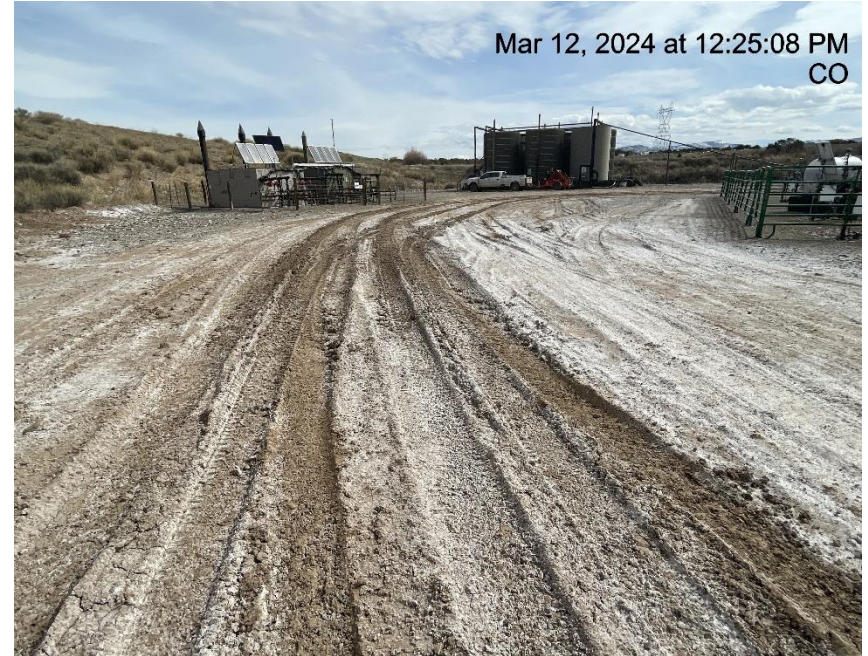
Photo # 9423 Lack of stabilization/compaction/insufficient tracking BMP's
