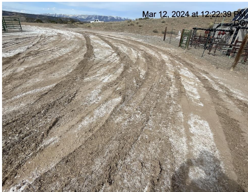
Photo # 9428 Lack of stabilization/compaction/insufficient tracking BMP's
