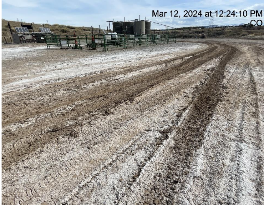
Photo # 9426 Lack of stabilization/compaction/insufficient tracking BMP's
