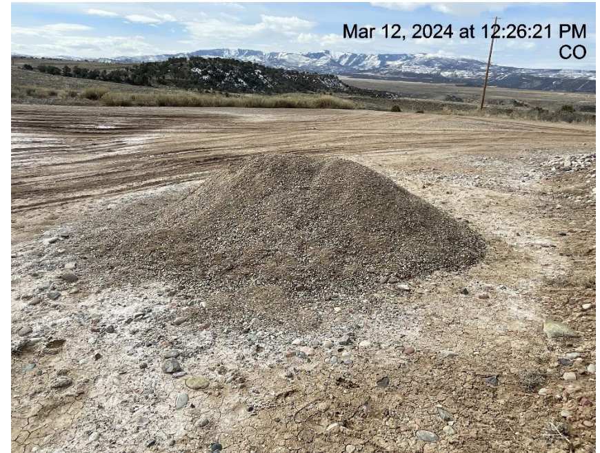
Photo # 9417 Stockpiled soils with no BMP's
