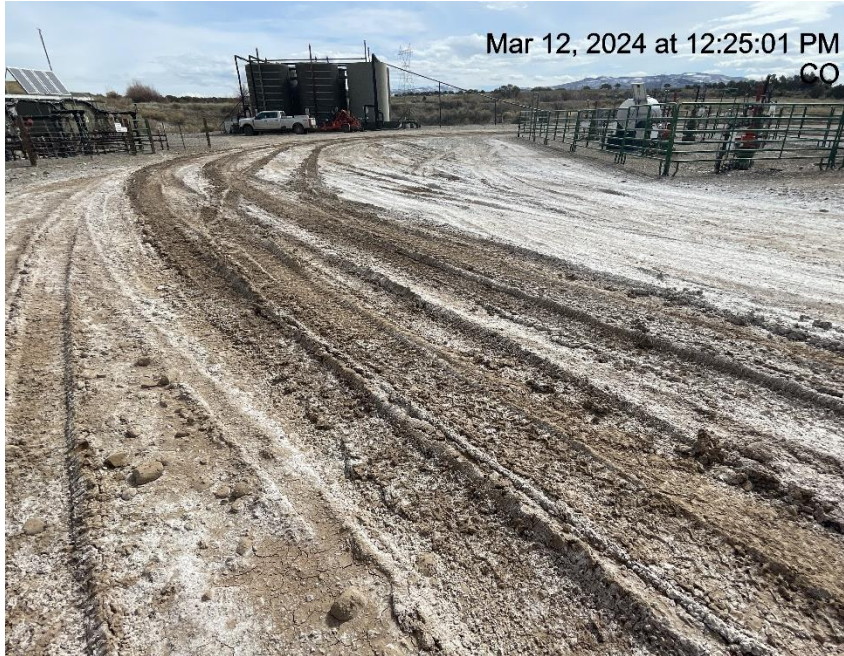
Photo # 9424 Lack of stabilization/compaction/insufficient tracking BMP's
