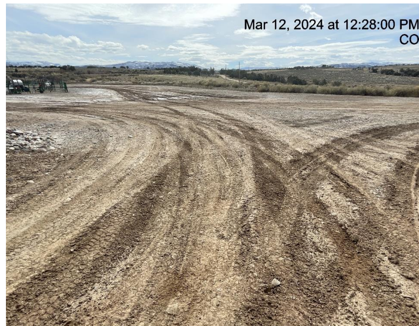
Photo # 9419 Lack of stabilization/compaction/insufficient tracking BMP's
