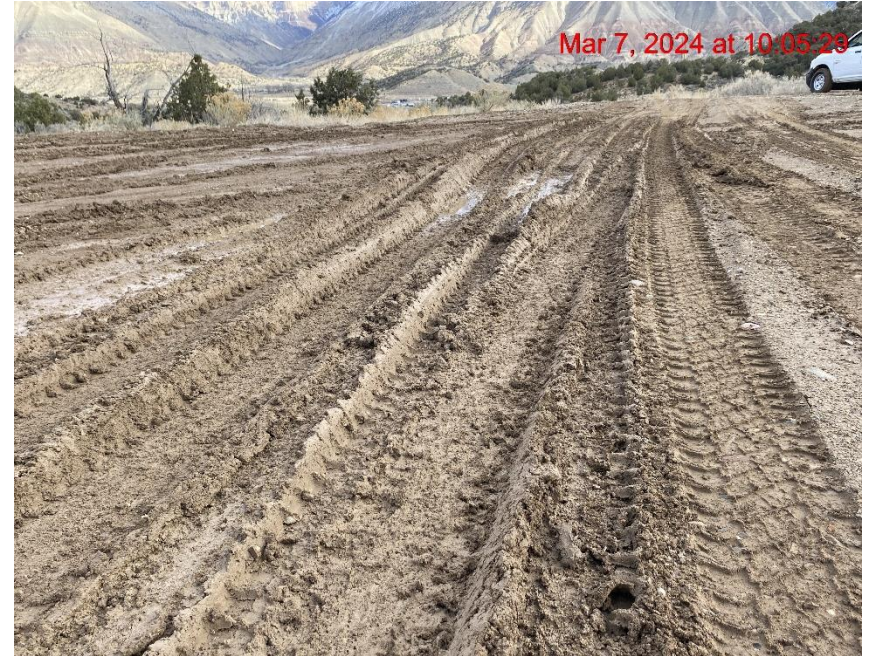
Lack of Stabilization – Photo #09750
