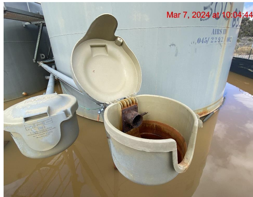
Open-Ended Load Line – Photo #09748
