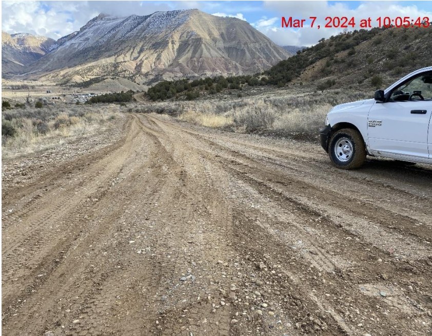
Insufficient Vehicle Tracking BMPs at Location Entrance/Exit – Photo #09751
