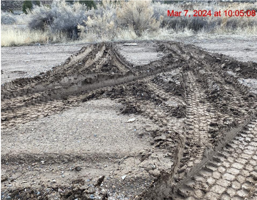
Lack of Stabilization – Photo #09749
