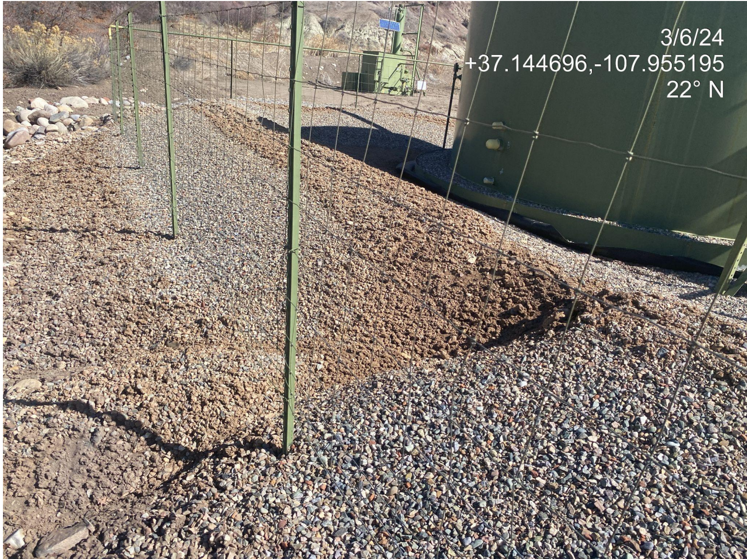
Photo 4. view of erosion impacting secondary containment around tanks.
