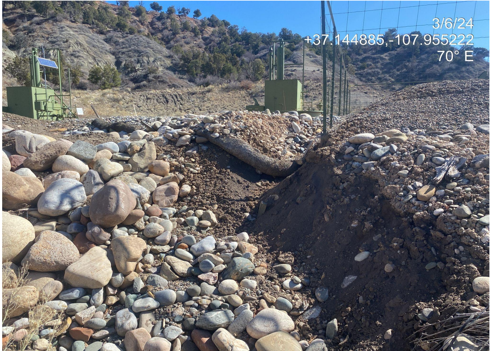
Photo 3. View of the persisting gully erosion and inadequate/failing storm water BMP issues observed in the western interim reclamation area.
