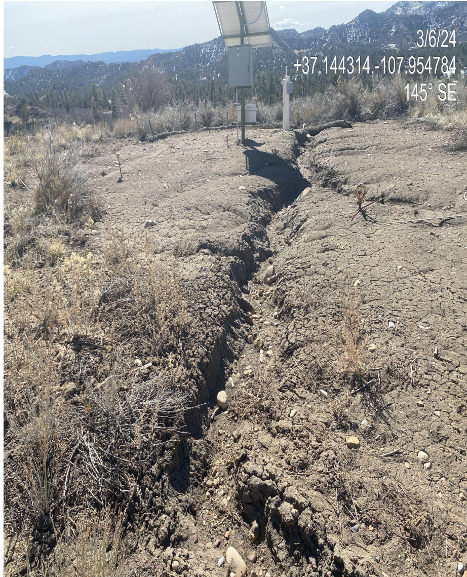
Photo 2. View of the persisting gully erosion and inadequate/failing storm water BMP issues observed in the southern interim reclamation area.
