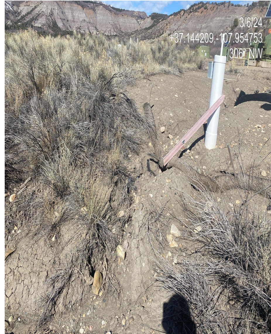
Photo 2. View of the persisting gully erosion and inadequate/failing storm water BMP issues observed in the southern interim reclamation area.
