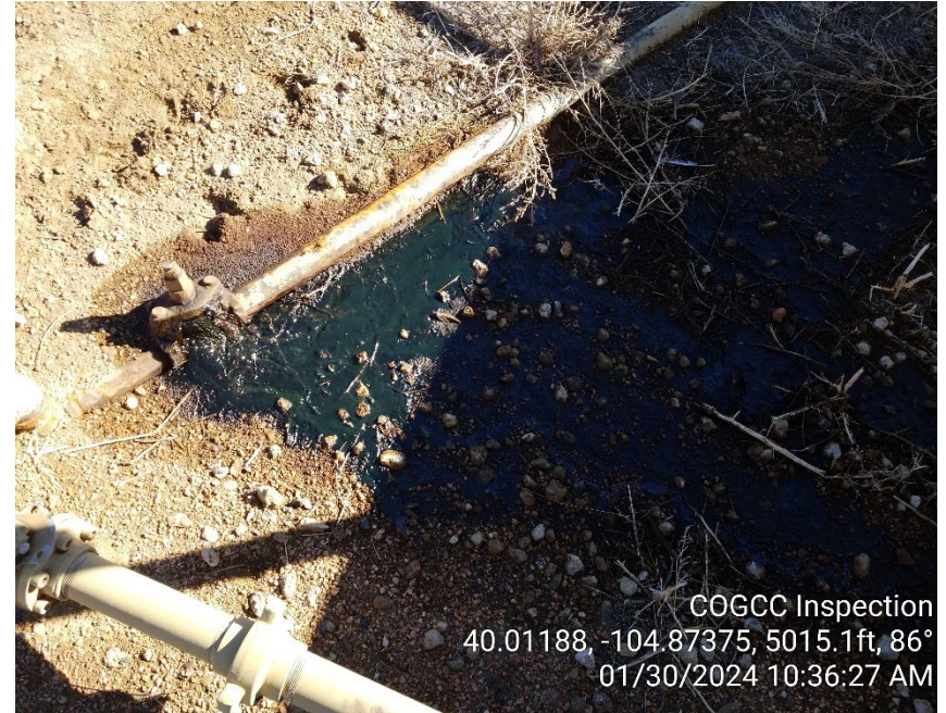
Photo 6 - Leak at separator
