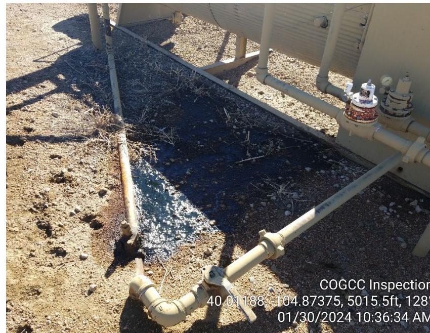
Photo 4 - Leak at separator
