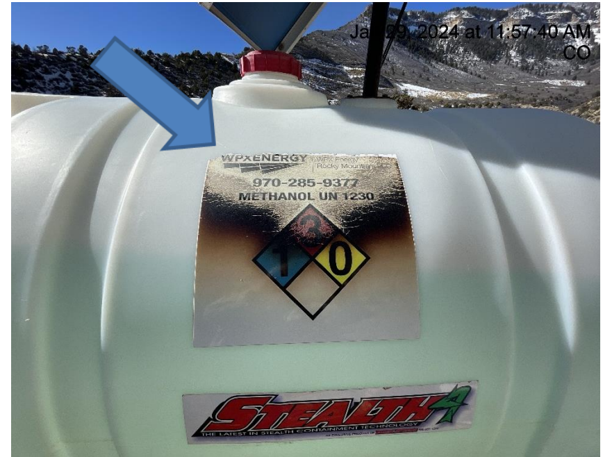
Photo # 4512 Chemical tank label has inaccurate info & lacks required info
