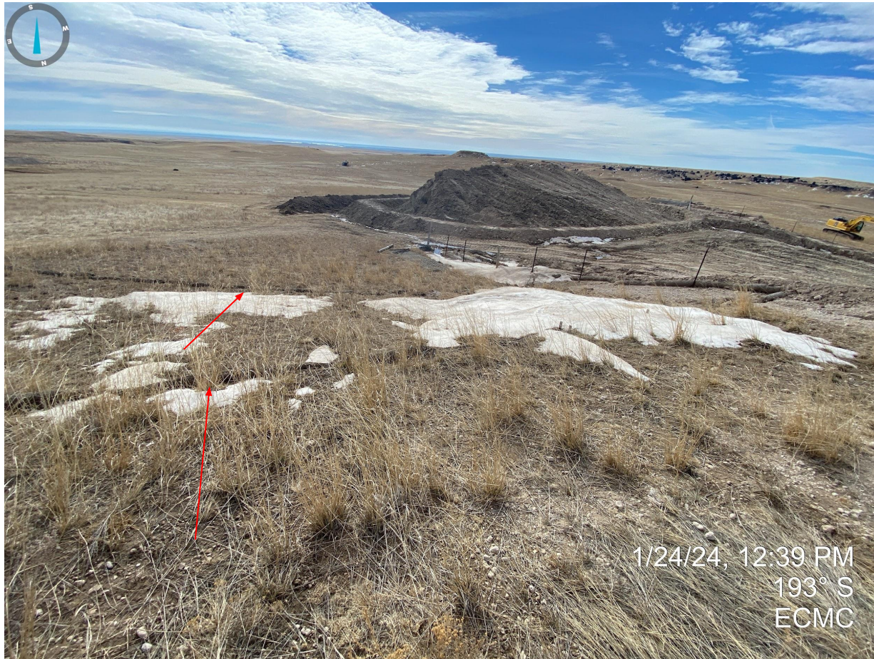
Photo 4. Taken south of pumpjack. Photo illustrates stockpile from pit in the background of the photo which is approximately 4,000 CY of material that has been placed outside of the location (approximately 0.5 of an acre of new disturbance). Straw wattle BMPs (red arrow) pictured in the foreground are degraded and now considered debris.
