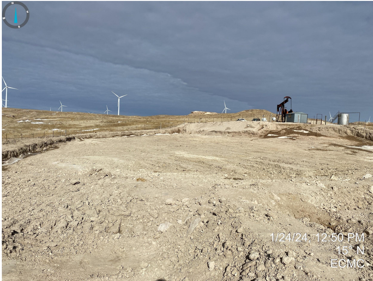
Photo 13. South side of excavated pit area. Soils do not appear to be properly stabilized as they have been left unconsolidated.
