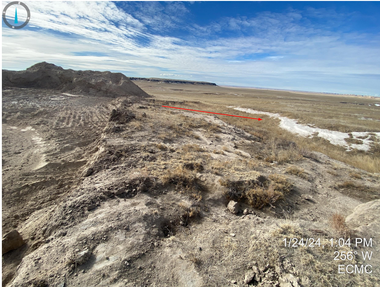
Photo 19. North side of salt kill excavation. No apparent stormwater control measures/BMPs observed that would prevent impacted material from the salt kill areas, or sediment laden stormwater, from entering adjacent drainage.
