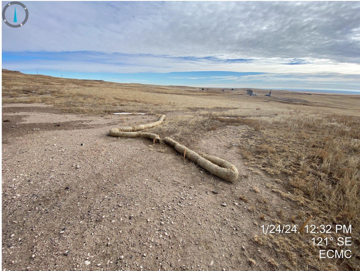
Photo 1. Taken near the vertical heater treater. Photo illustrates that straw wattles are not properly installed and bare/exposed soils are not properly stabilized.
