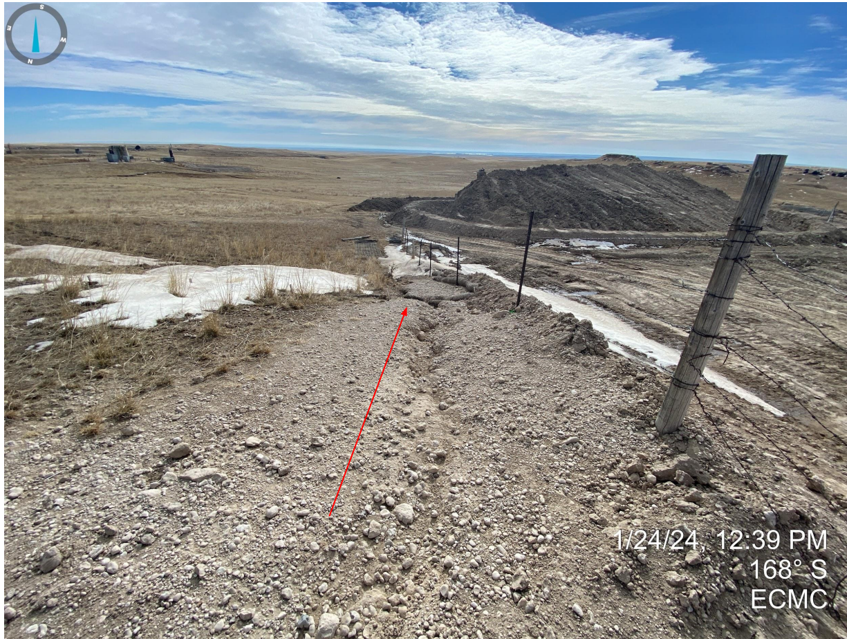
Photo 5. Erosion degradation on the east side of the pit. No stormwater control measures observed.
