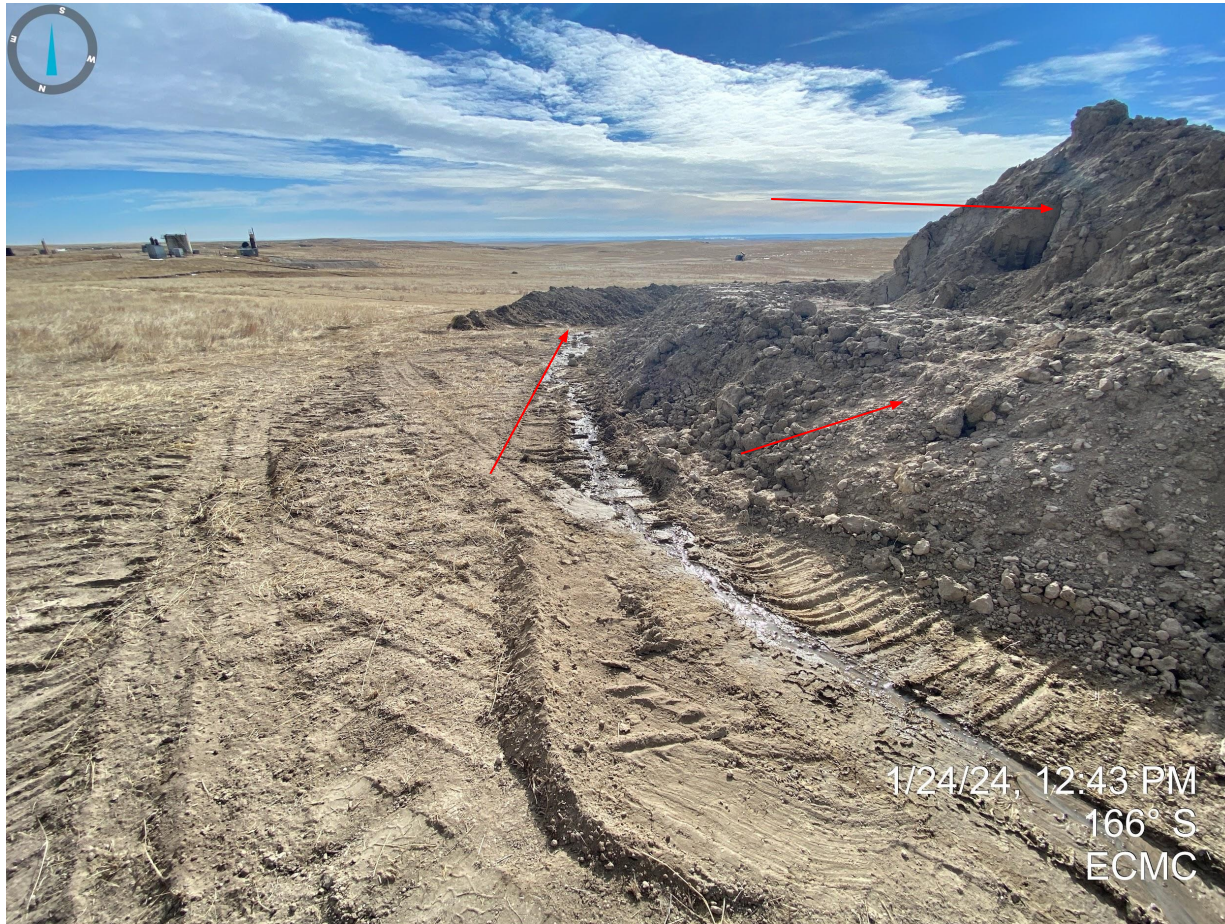
Photo 7. Northeast side of stockpiled pit soils. Photo illustrates that both the stockpile and berms have been left unconsolidated. Unconsolidated materials can become a potential pollution source as it is not properly stabilized. Also pictured, stormwater running off location into berms.
