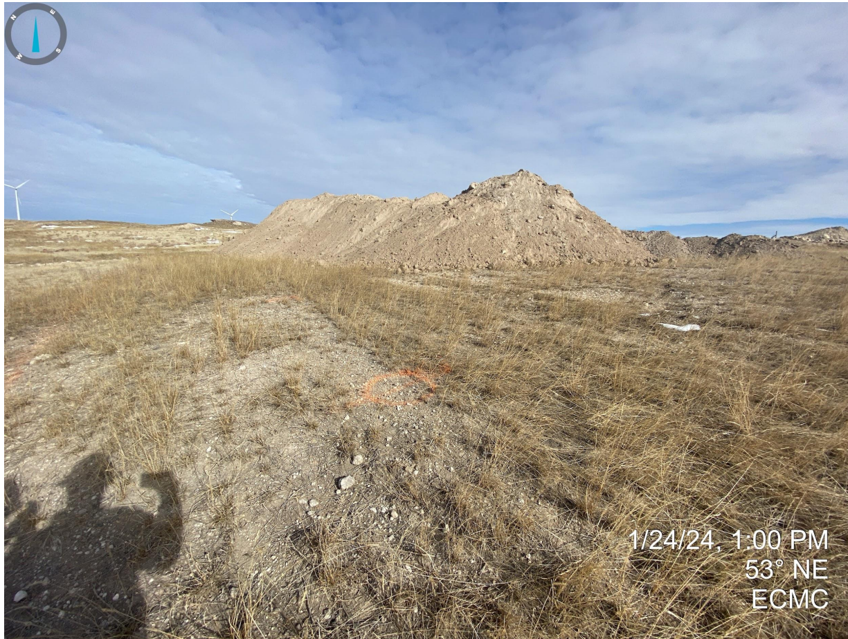
Photo 15. Southwest of the western salt kill excavation. No apparent stormwater control measures/BMPs were observed at the time of this inspection. Stockpiled material is not properly stabilized as it has been left unconsolidated.
