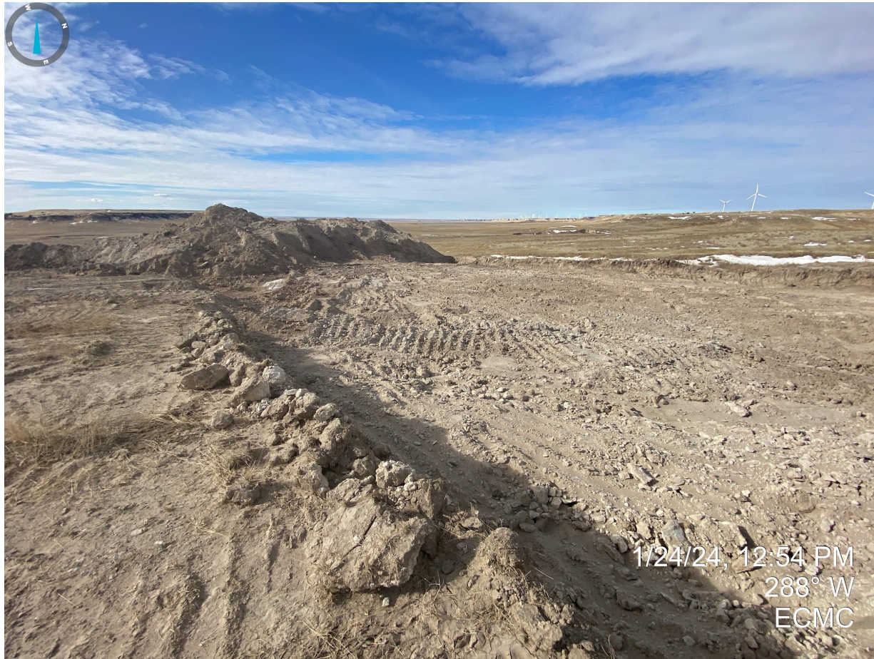
Photo 14. Excavated area west of the pit is approximately 0.5 acre in size and the stockpile is approximately 4,000 CY. Operator will need to submit an updated Form 2A as this disturbance is occurring outside of the original disturbance area. Soils do not appear to be properly stabilized from wind and water erosion.
