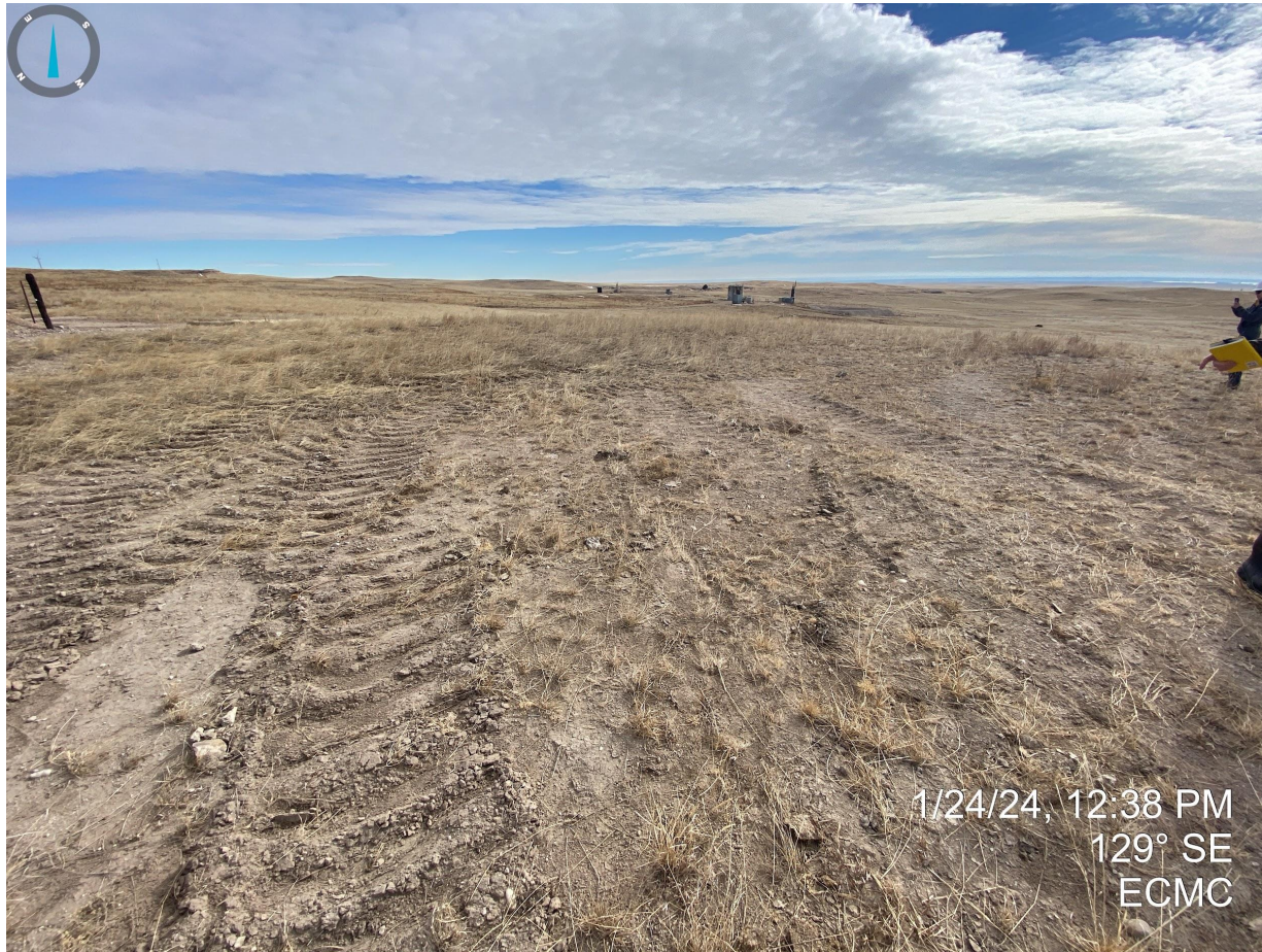
Photo 3. Taken between the vertical heater treater and pumpjack. Photo illustrates that the bulldozer has been removed from the location, and any disturbances resulting in bare/exposed or unstabilized soils will need to be properly stabilized with appropriate BMPs.
