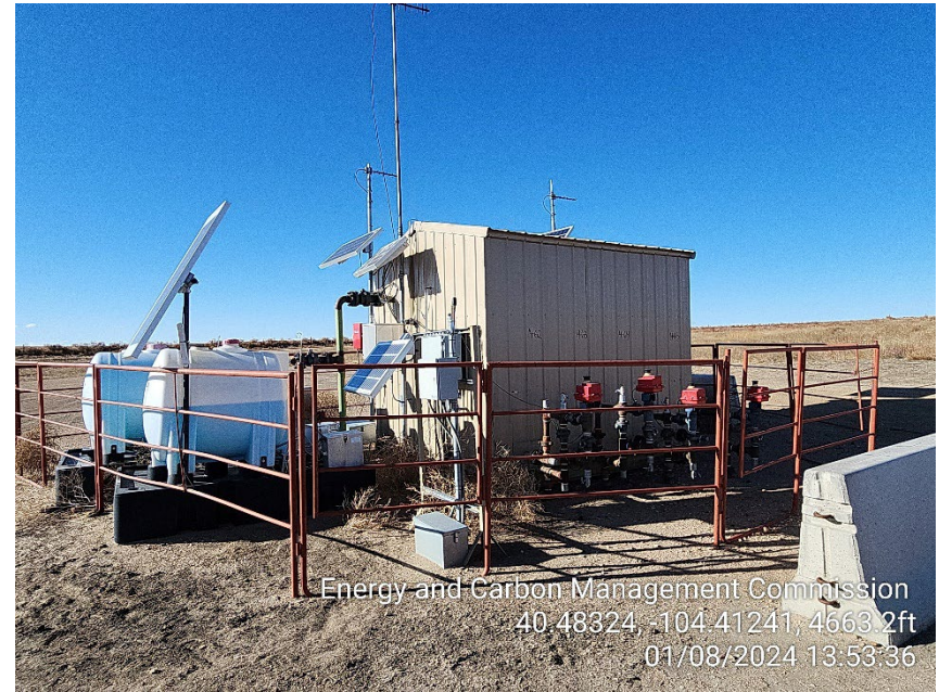
Photo 4 – Gas Lift Injection Meter House
