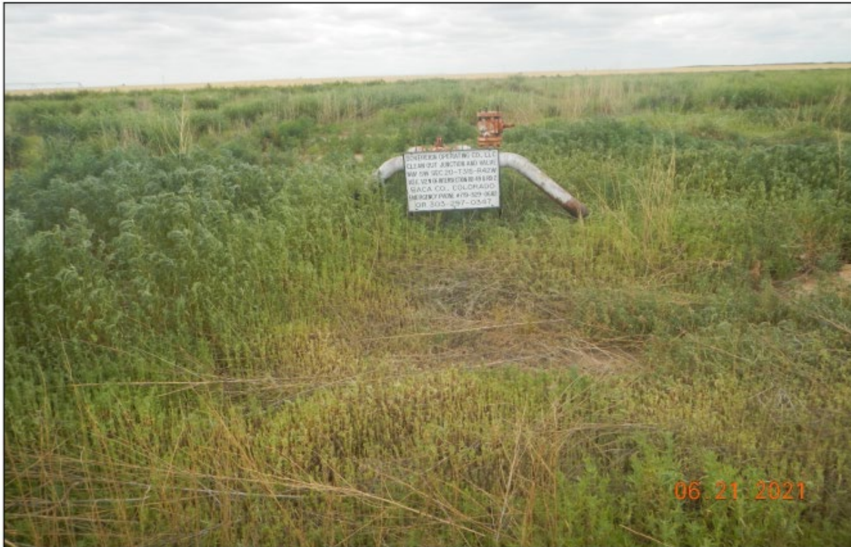
Photo 7. There is a cleanout junction 1850 ft. north of the pipeline which is associated with the former gas compressor station and must be removed. Photo taken from previous inspection.
