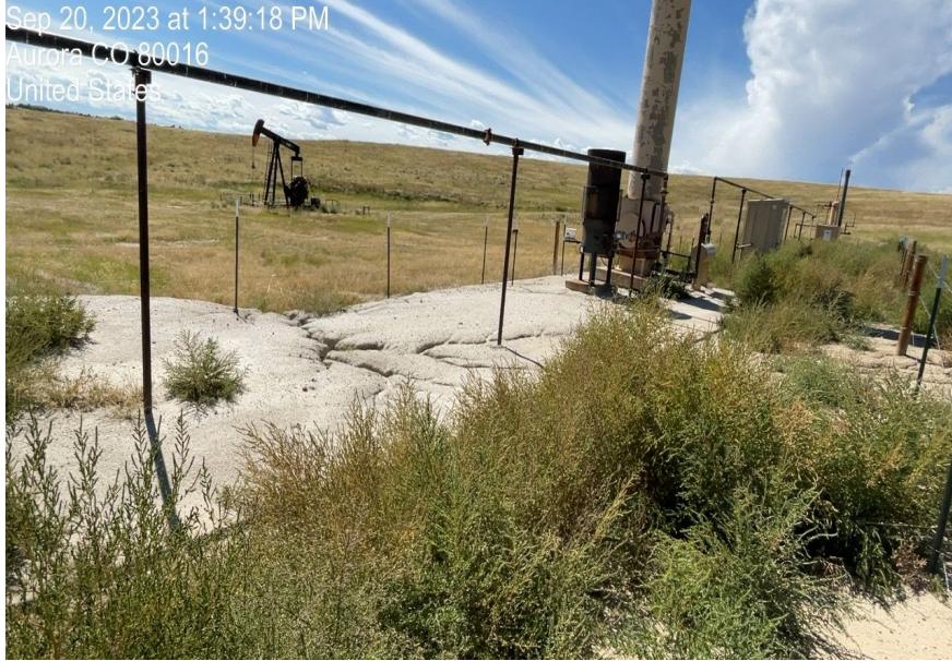
Photo 5. Photo of weeds (kosha & russian thistle) and erosion around burner on tank battery. Photo taken facing northwest.
