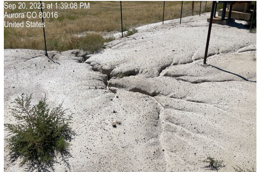
Photo 4. Photo of gulying from stormwater near bunner on tank battery pad. Photo taken facing northwest.
