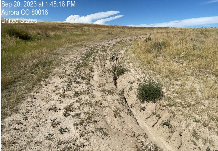
Photo 11. Photo taken of access road to wellhead, stormwater erosion causing deep gulying. Photo taken facing northeast.
