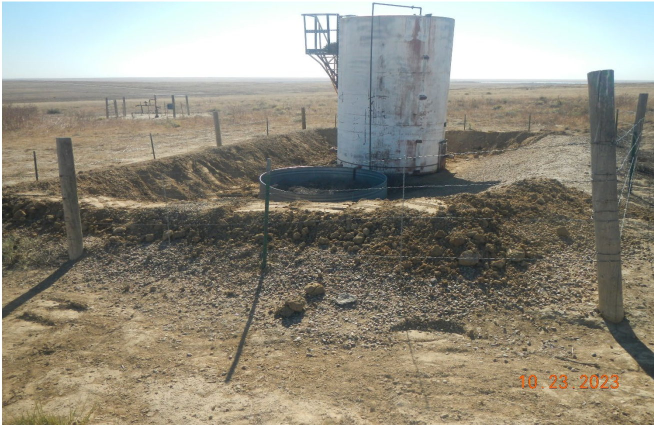
Photo 2. Facing southeast toward the tank battery. The secondary containment has been built up higher.
