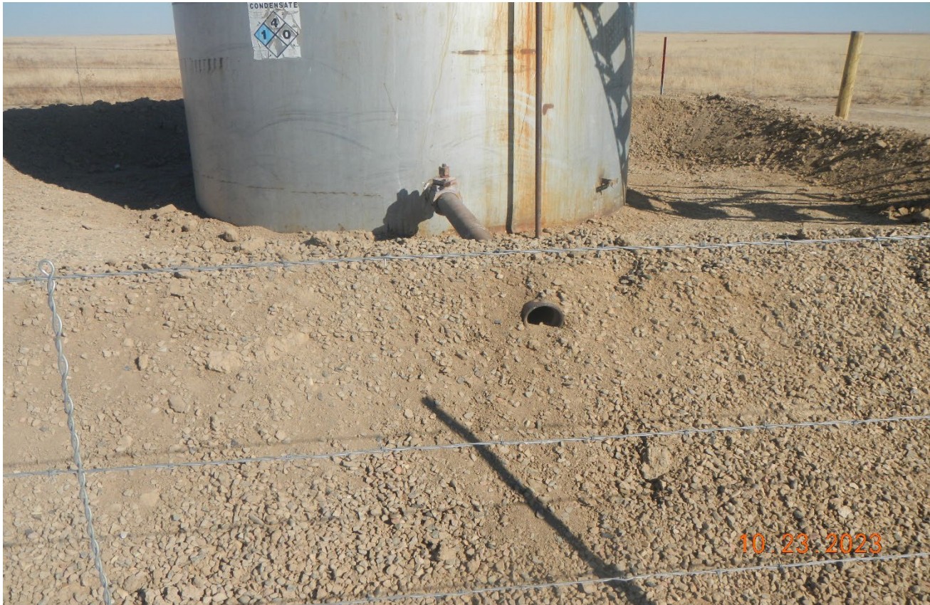
Photo 4. This pipe is exposed on the outside of the tank battery and is not contained inside containment,.
