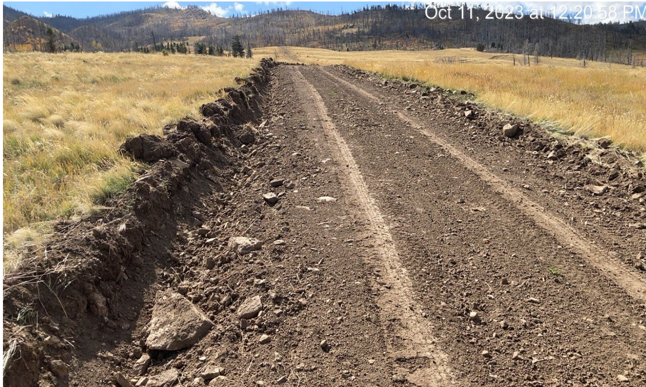
Photo 2. Facing southwest along the access road. The road has recently been graded however, no other BMP's have been installed.
