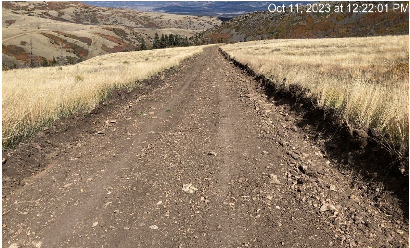
Photo 3. Facing northeast back down the access road. Grading activities as the only BMP is not sufficient to stabilize the road and prevent stormwater erosion issues of the road.
