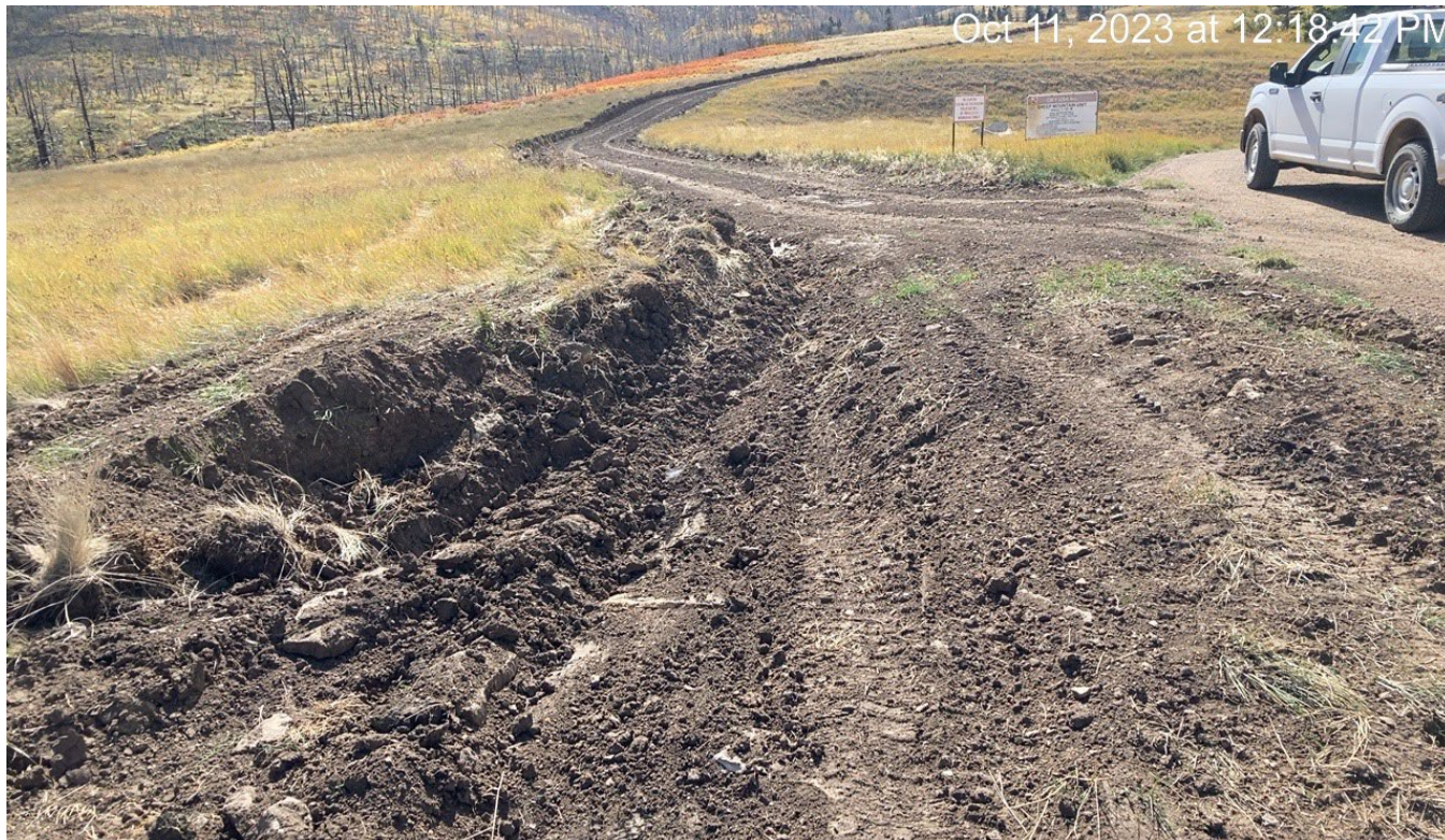
Photo 1. Facing southwest along the access road near the SMU #1-12-B . This area was bladed and sediment was pushed further out creating disturbance. Grading activities as the only BMP is not sufficient to stabilize the road.
