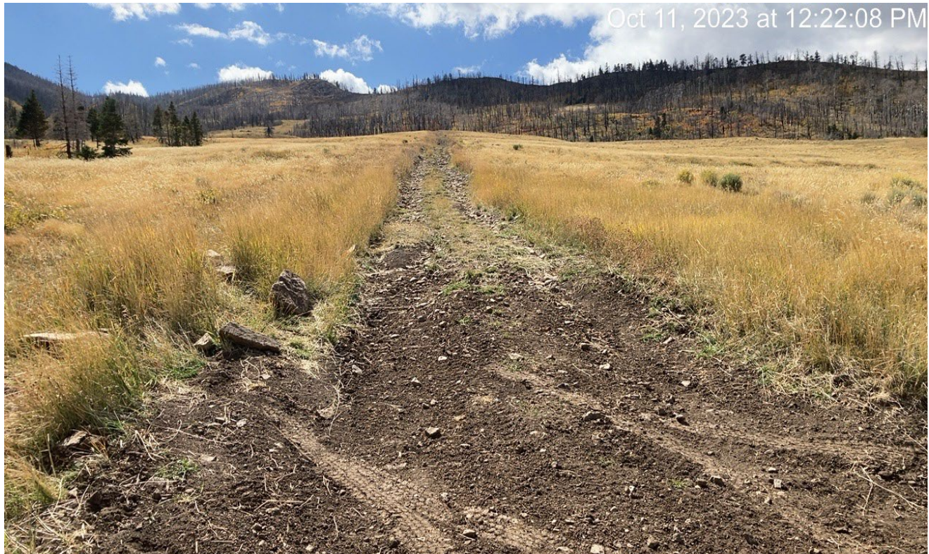
Photo 4. Facing southwest along the access road. Grading of the road stopped at this point and the remainder of the road remains eroded with insufficient BMP maintenance.
