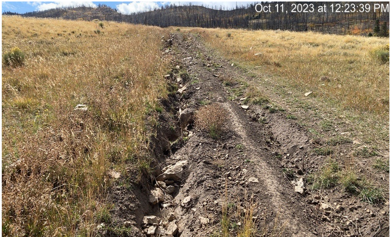
Photo 5. Facing southwest further along the access road. There are areas of erosion occurring which need to be repaired and stabilized.
