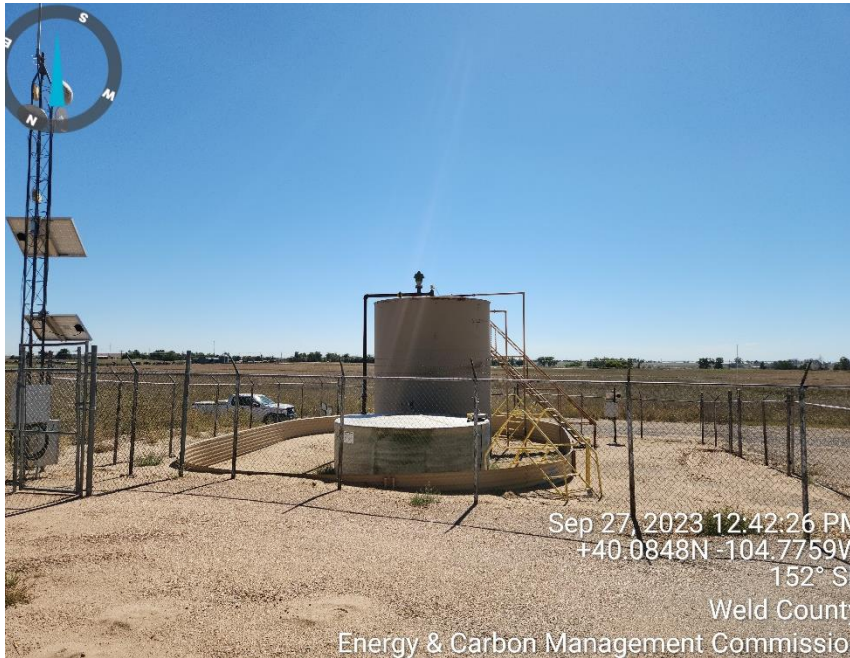
Photo 7 tank battery
