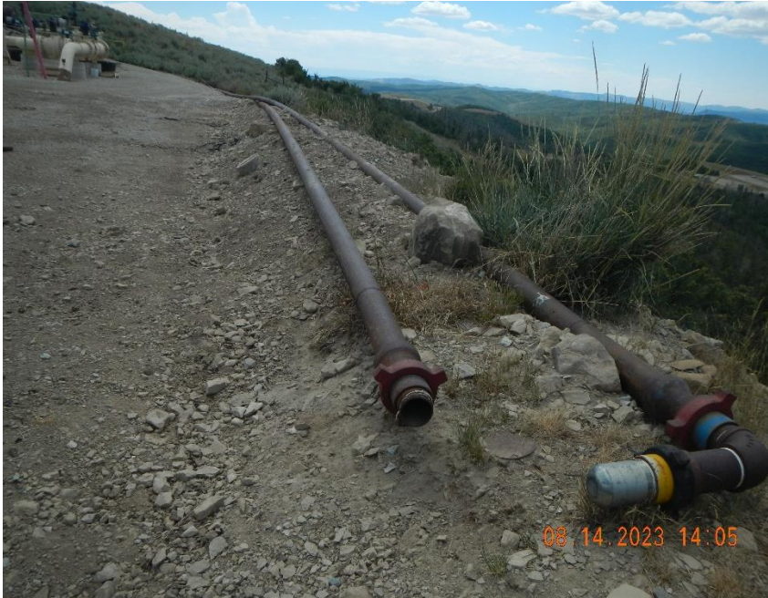
1 of the south flowlines is open ended, the plug is on the ground near the line.
