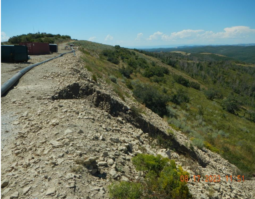
Breach of berm and erosion of hillside along the west edge of location.
