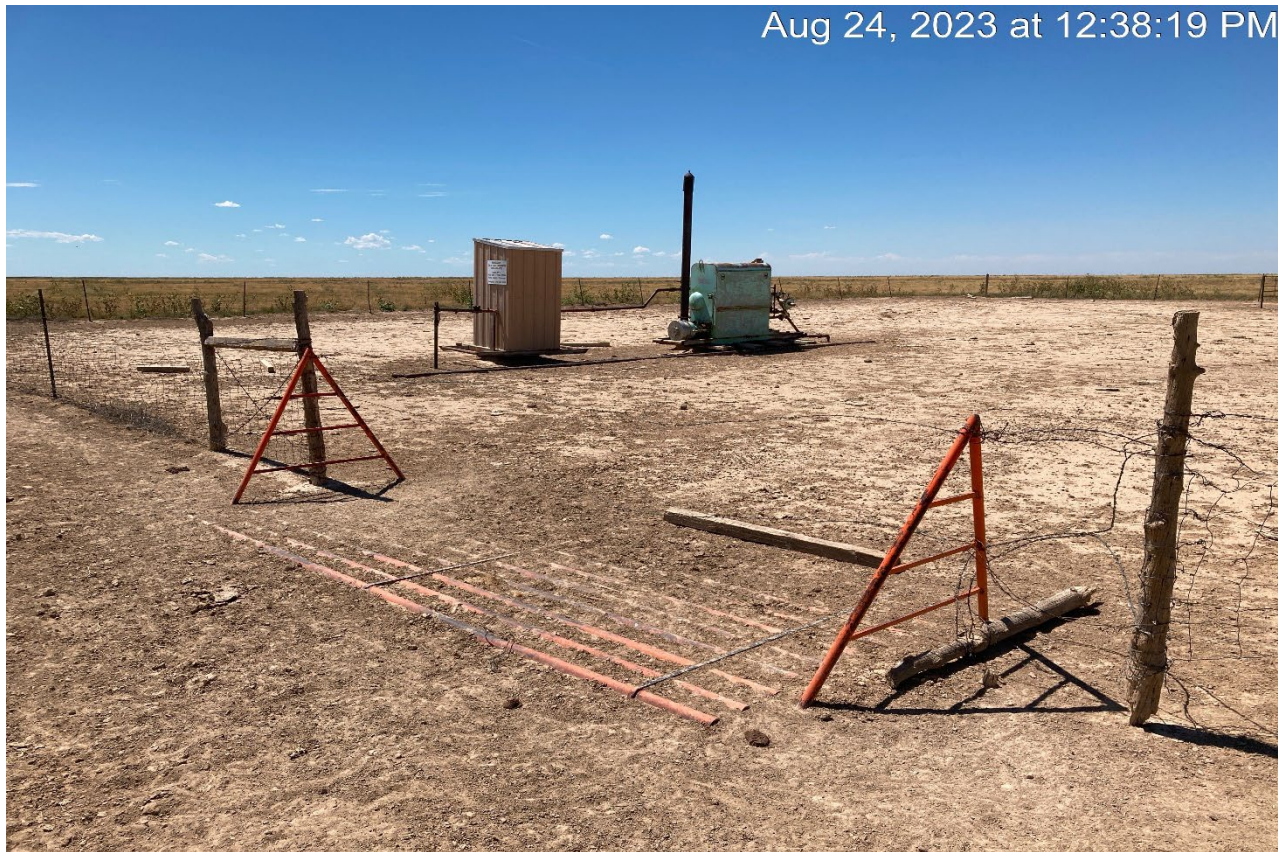
Photo 1. Facing southwest toward the location. The cattlegurd entering the location is filled in with sediment and needs to be maintained.
