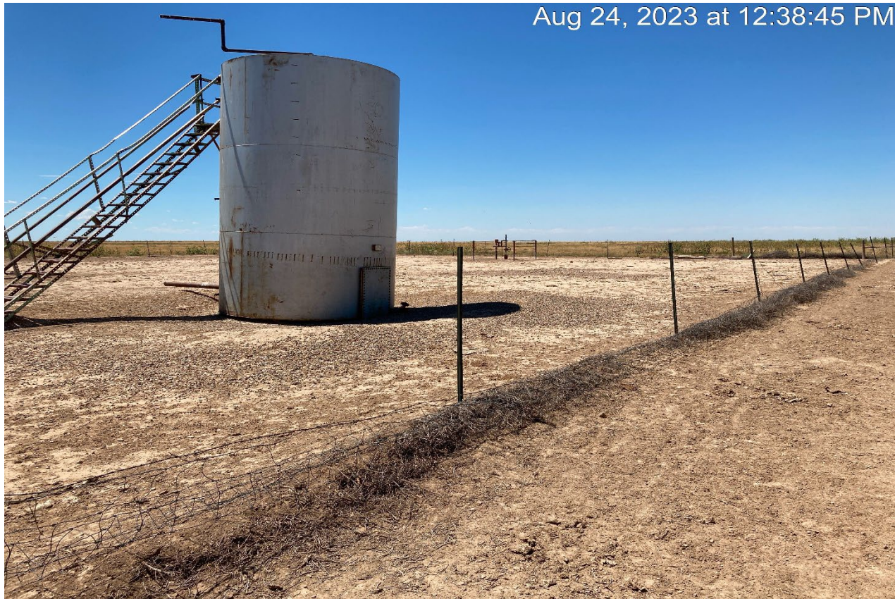
Photo 2. The secondary containment at the tank is insufficient to contain a spill.
