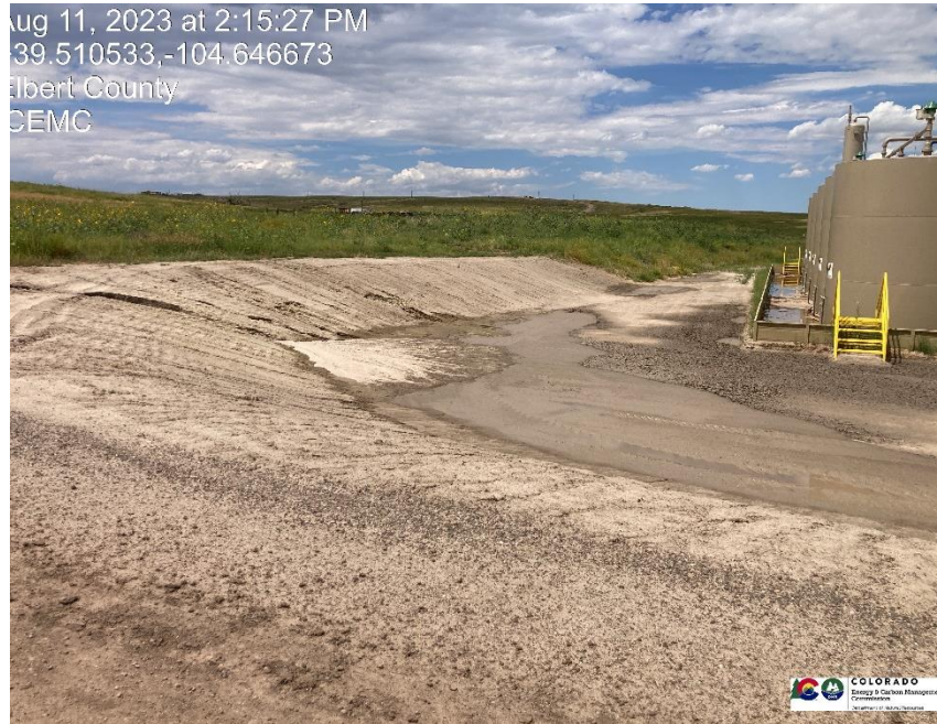
Pic 1 Stormwater control measures failure.
