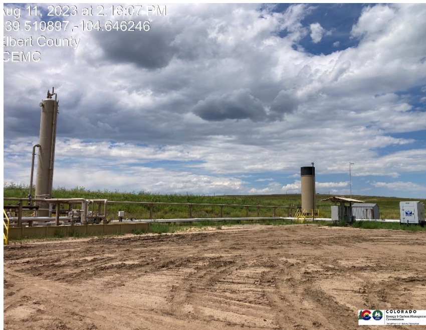
Pic 3 VRT, VRU, ECD, generators
