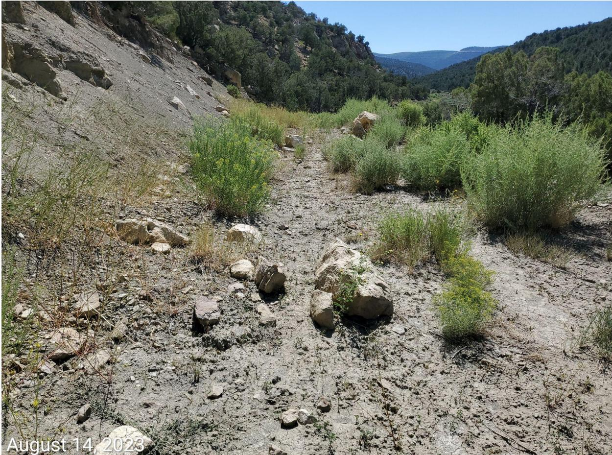
**Photo 9:** Photo example showing erosion degradation along access road. Stormwater and erosion control measures remain inadequate. Access road has not been decompacted, recontoured, regraded and reclaimed in accordance with 1004 Rules.
