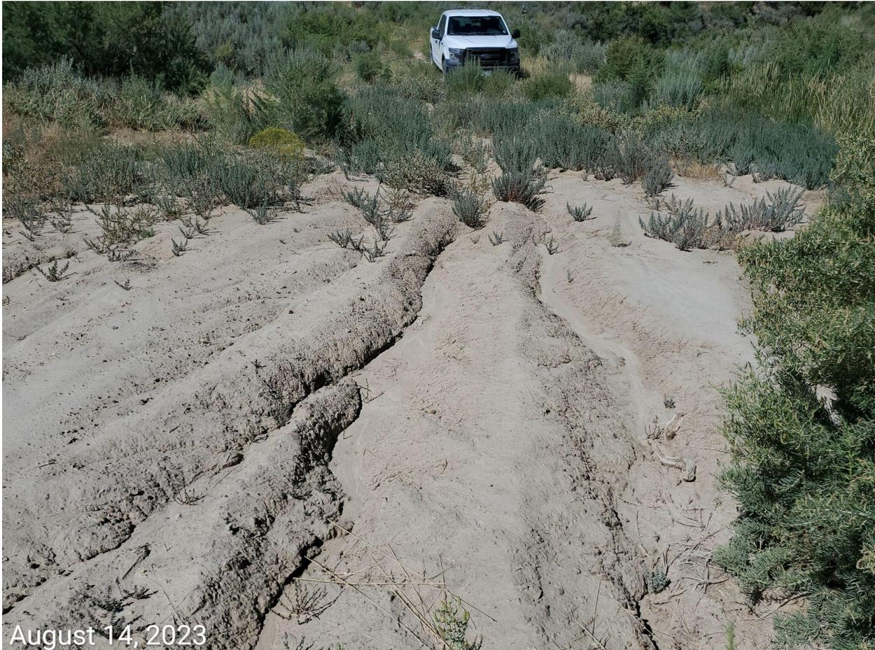
**Photo 14:** Photo example showing erosion degradation along access road. Stormwater and erosion control measures remain inadequate. Access road has not been decompacted, recontoured, regraded and reclaimed in accordance with 1004 Rules. Photo also shows Halogeton establishment on access road.
