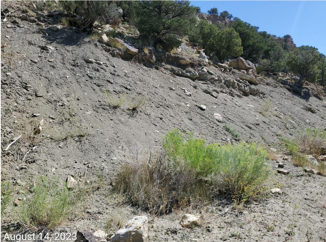
**Photo 8:** Photo example showing erosion degradation along access road. Stormwater and erosion control measures remain inadequate. Access road has not been decompacted, recontoured, regraded and reclaimed in accordance with 1004 Rules.
