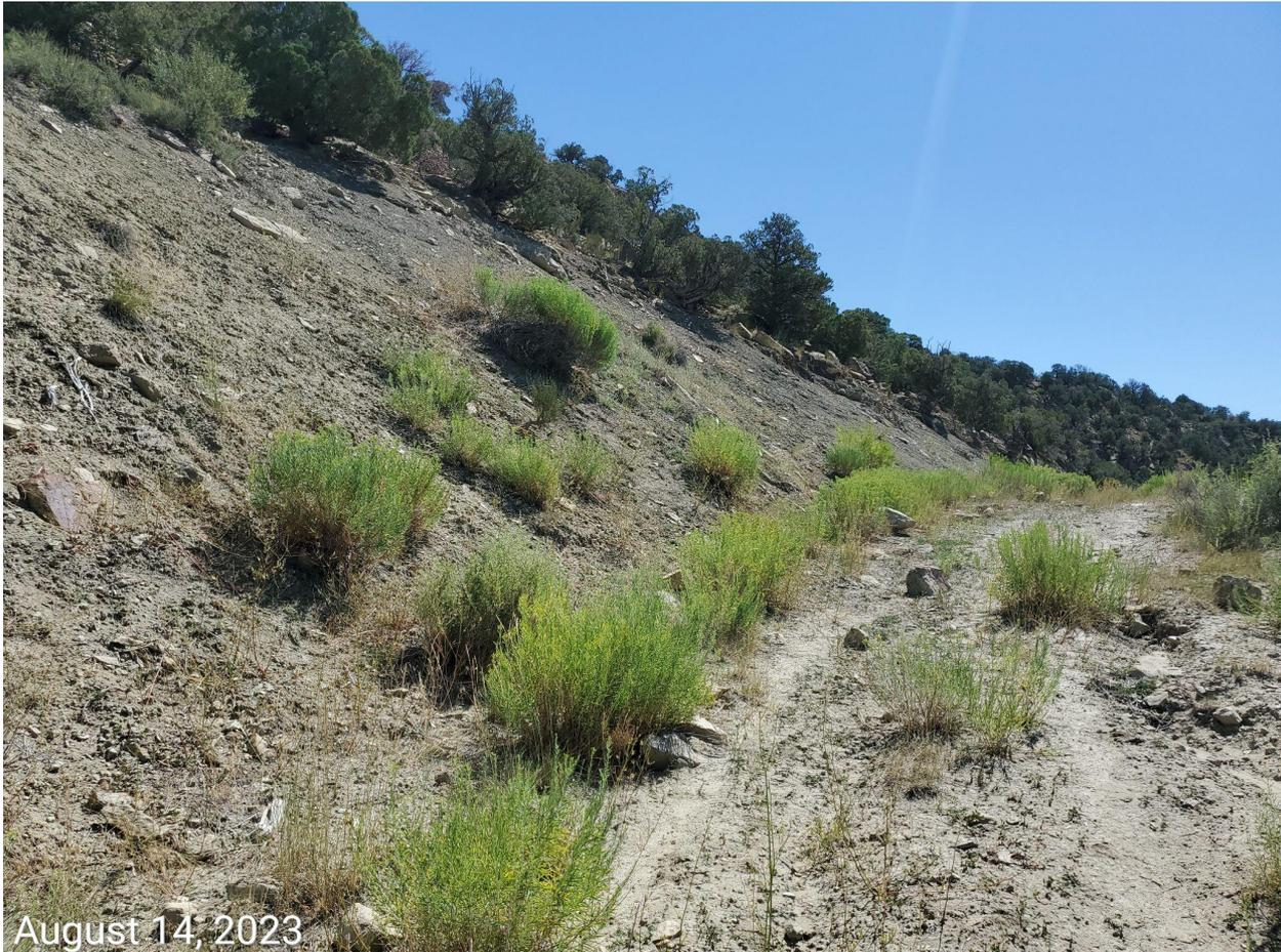
**Photo 6:** Photo example showing erosion degradation along access road. Stormwater and erosion control measures remain inadequate. Access road has not been decompacted, recontoured, regraded and reclaimed in accordance with 1004 Rules.
