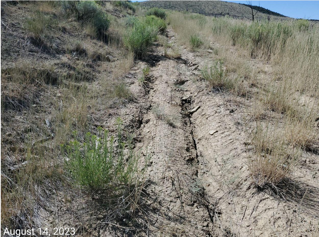
**Photo 12:** Photo example showing erosion degradation along access road. Stormwater and erosion control measures remain inadequate. Access road has not been decompacted, recontoured, regraded and reclaimed in accordance with 1004 Rules.
