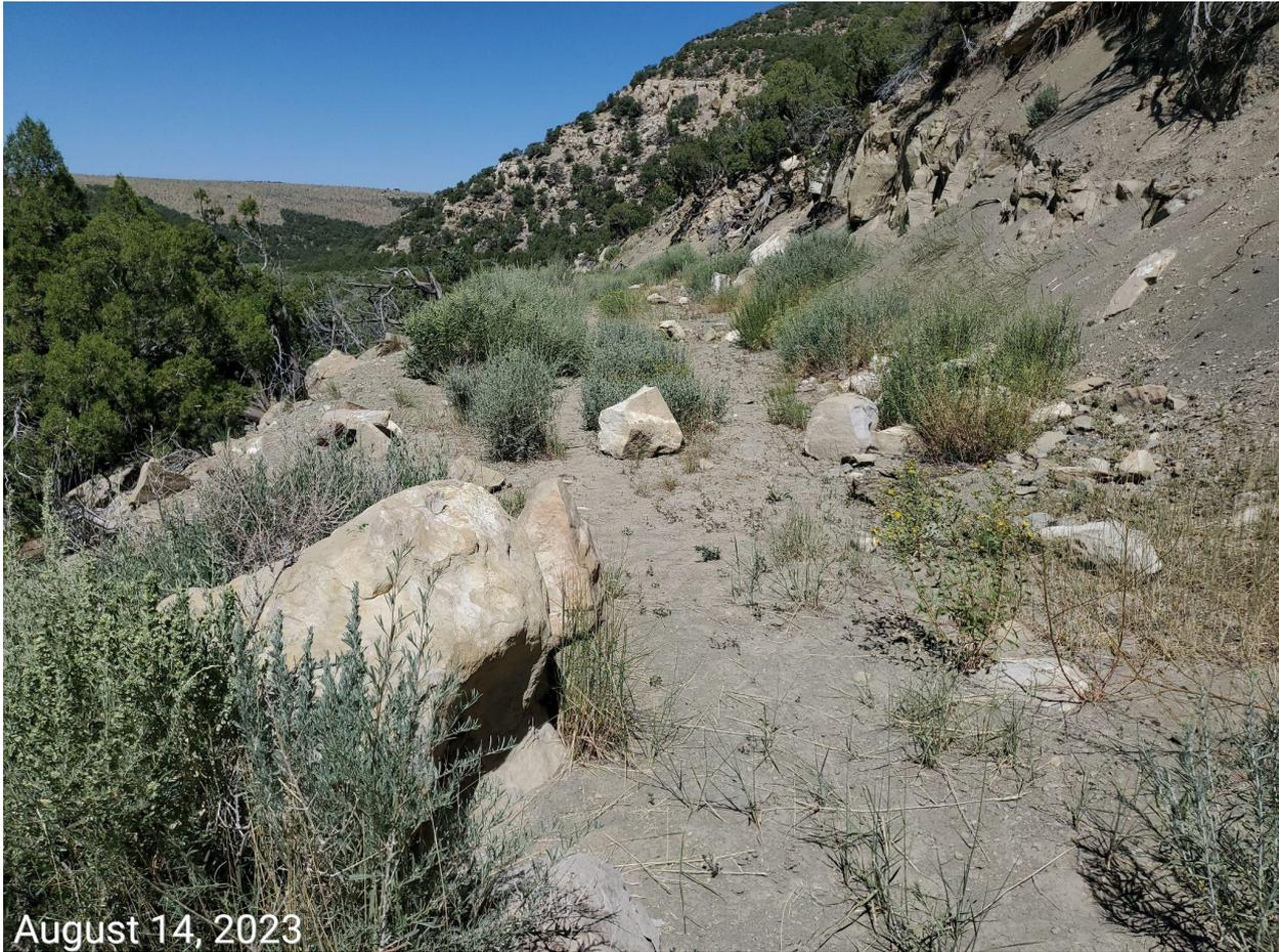
**Photo 10:** Photo example showing erosion degradation along access road. Stormwater and erosion control measures remain inadequate. Access road has not been decompacted, recontoured, regraded and reclaimed in accordance with 1004 Rules.
