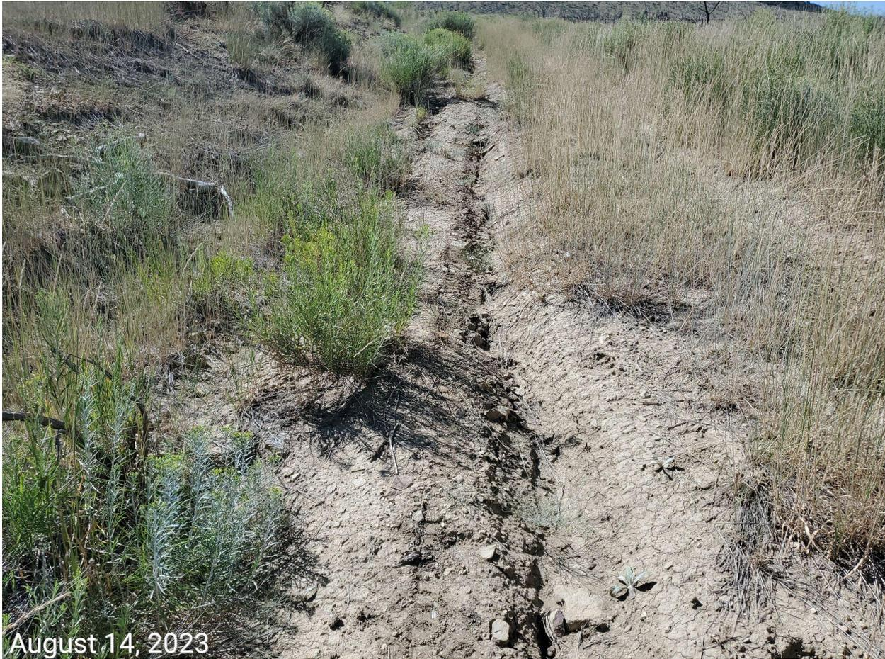
**Photo 11:** Photo example showing erosion degradation along access road. Stormwater and erosion control measures remain inadequate. Access road has not been decompacted, recontoured, regraded and reclaimed in accordance with 1004 Rules.
