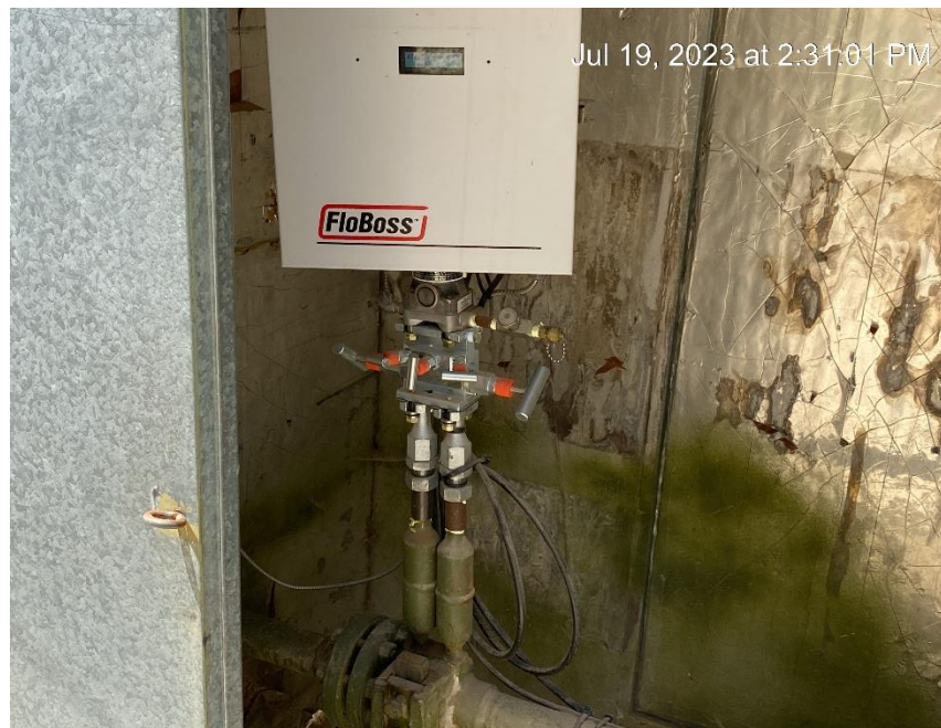
No visible display of gas meter calibration
