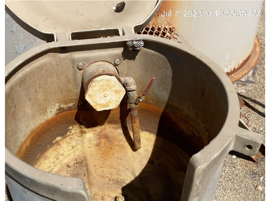
Open end loadline. Valve open.
