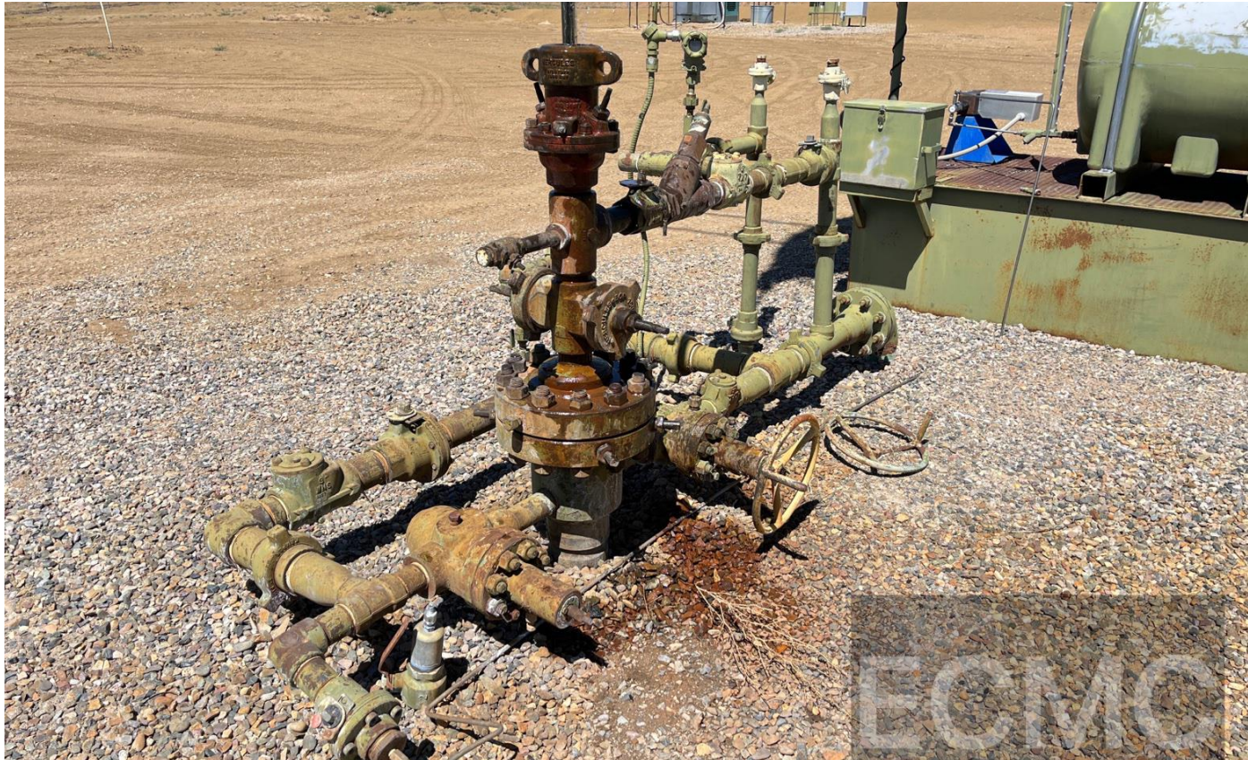
Photo #2. View of the wellhead assembly and impacted material.
