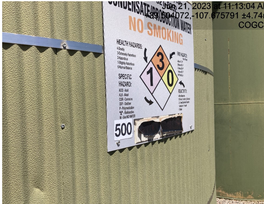
Sicker added to tank from last inspection is lacking BBLS
