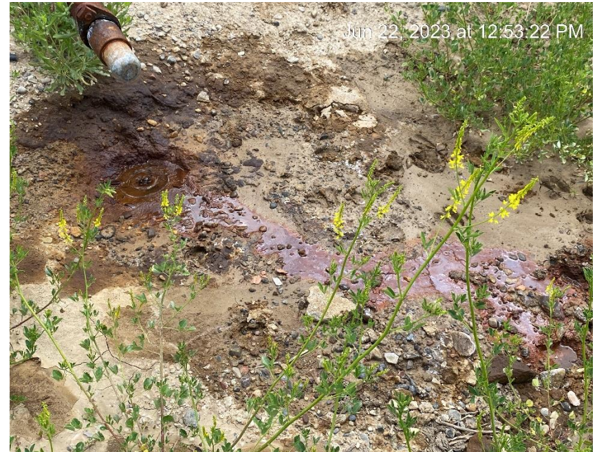
Steady drip from leaking line
