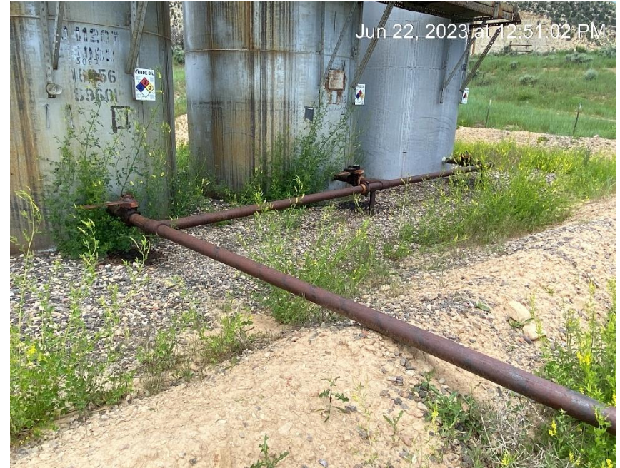
Valve leaks. Stained soils.
