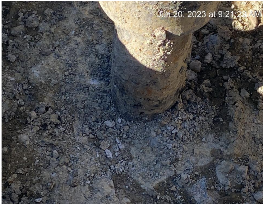
Cellar ring excavated to top of conductor (cement)
