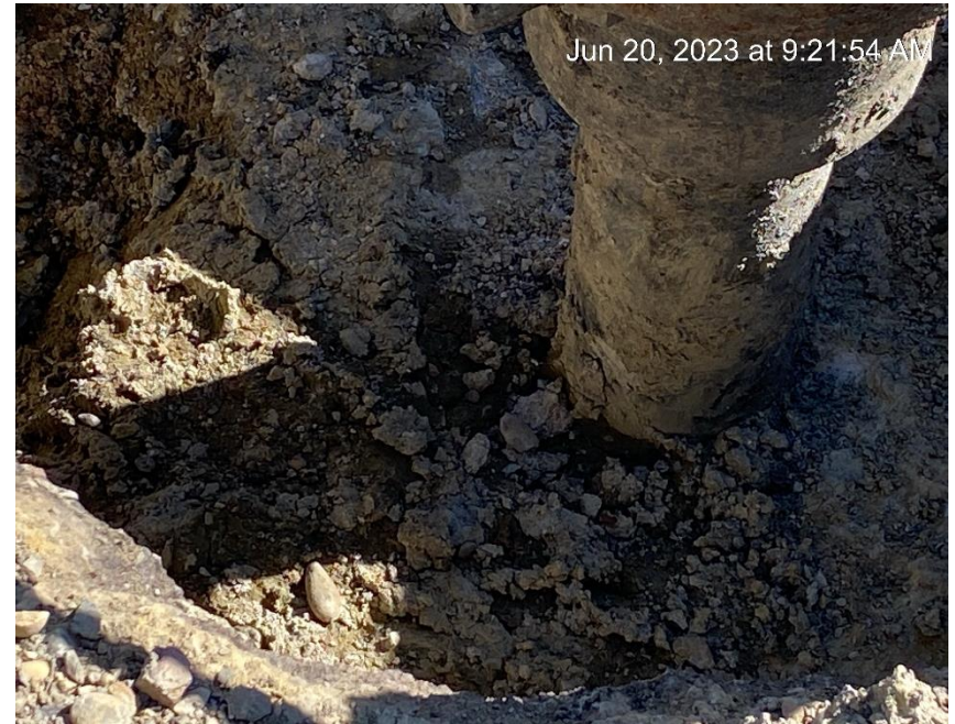
Cellar ring excavated to top of conductor (cement)
