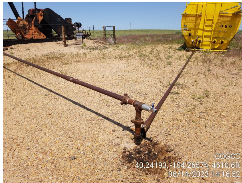
Photo 2 – Stained Soil at Hardline Connection
