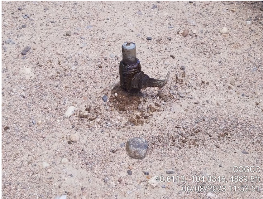
Photo 3 – Stained Soil and Unmarked Riser
