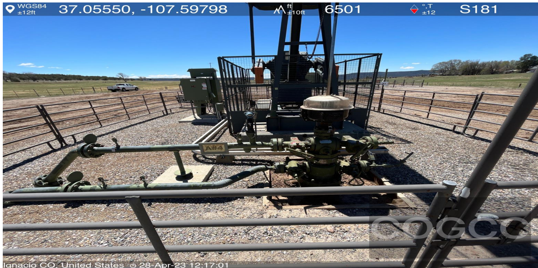
Photo #2. Wellhead assembly.
