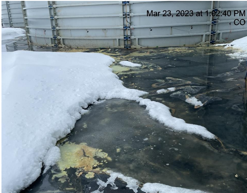
Photo # 2998 E & P waste in secondary containment
