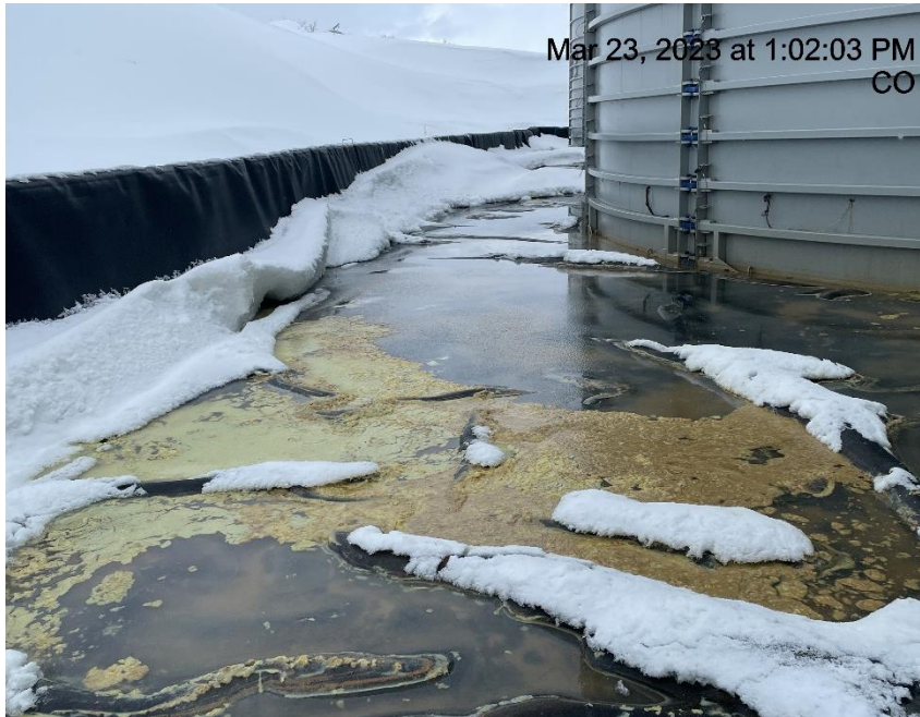
Photo # 2996 E & P waste in secondary containment
