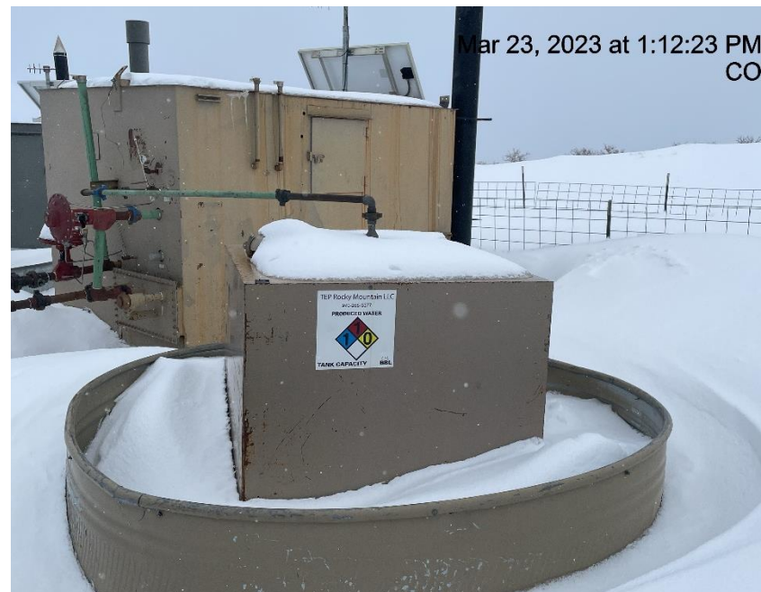
Photo # 3008 Tank label missing required info
