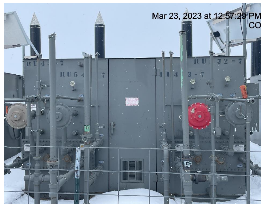
Photo # 2989 Meter calibration info not conspicuously posted
