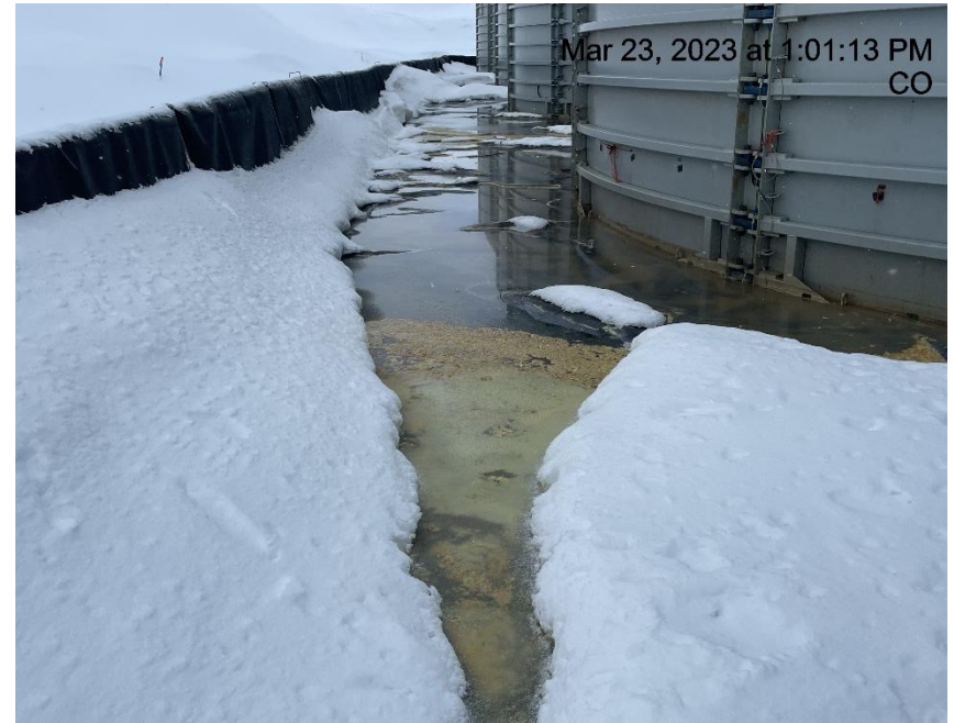
Photo # 2993 E & P waste in secondary containment
