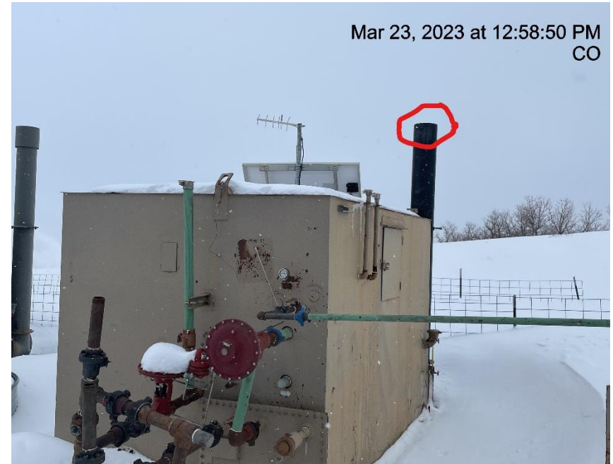
Photo # 3010 Production unit missing bird protection on burner stack
