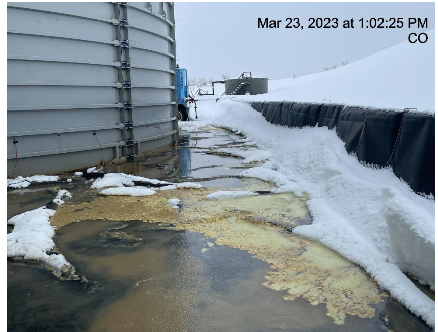
Photo # 2997 E & P waste in secondary containment
