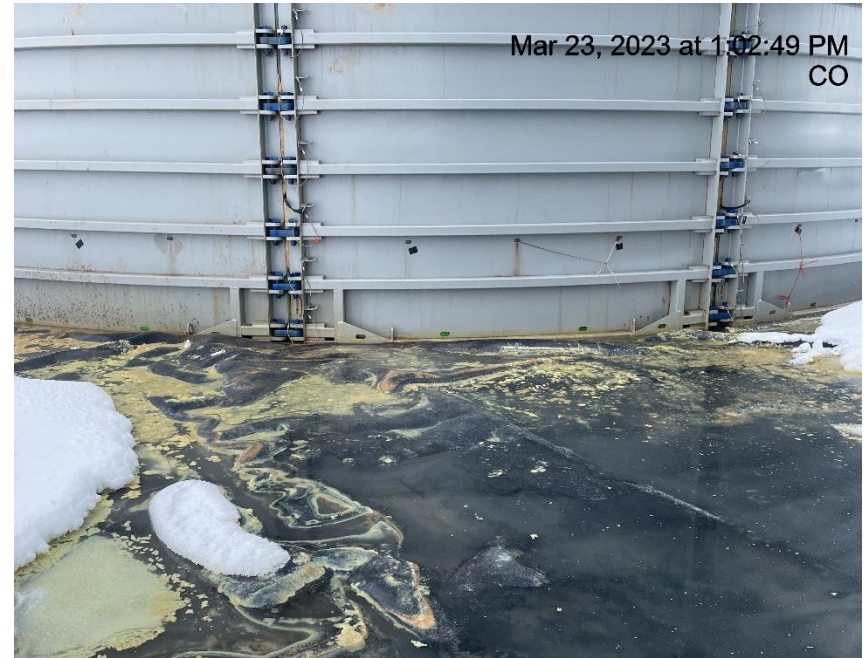
Photo # 2999 E & P waste in secondary containment
