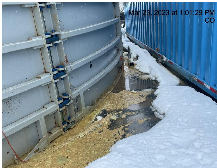
Photo # 2994 E & P waste in secondary containment
