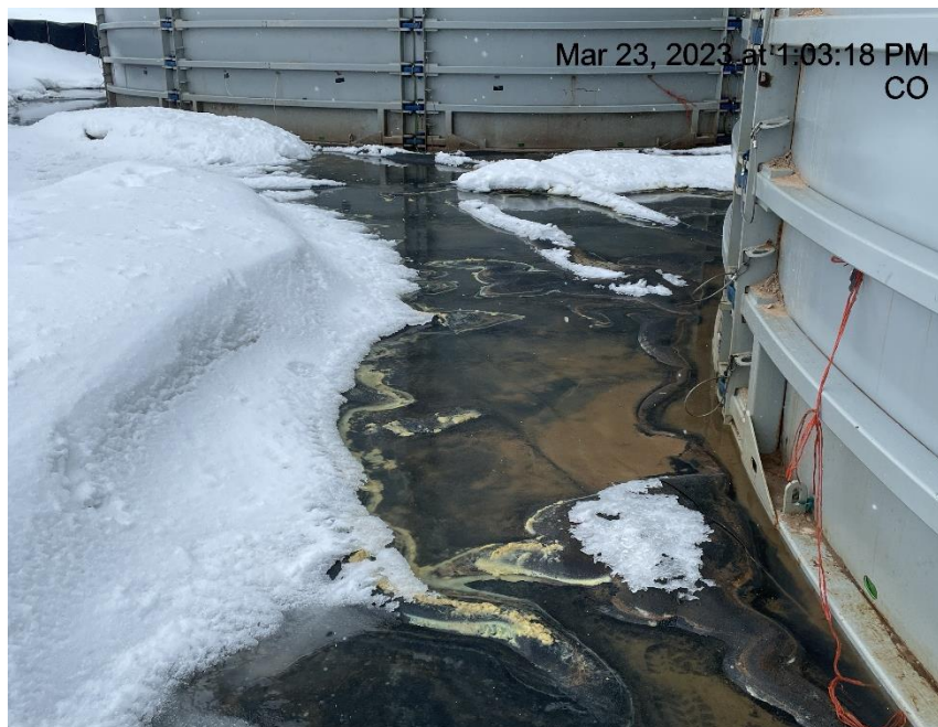
Photo # 3000 E & P waste in secondary containment
