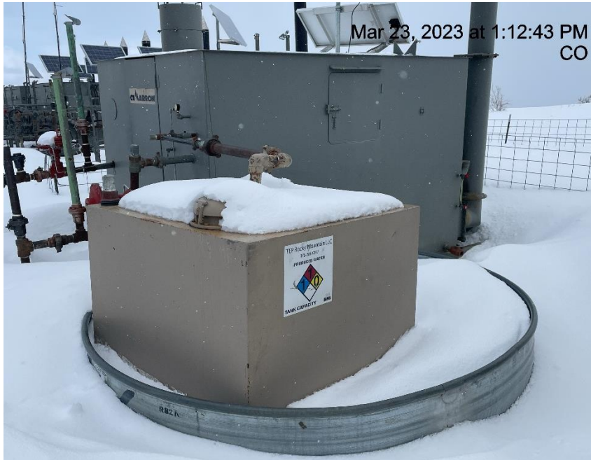
Photo # 3009 Tank label missing required info
