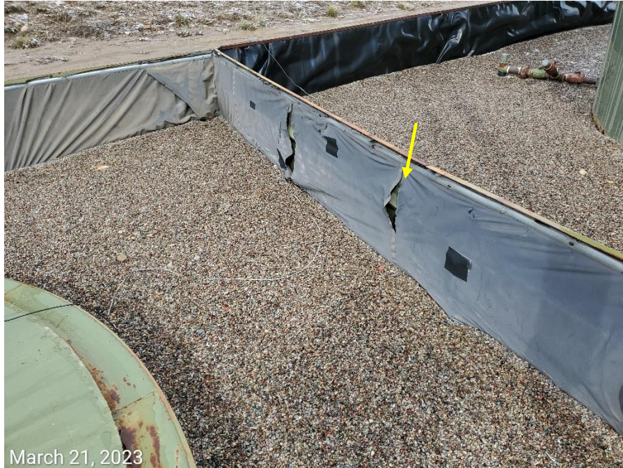
Photo 6: Photos show liner integrity, and tank labeling corrective actions have not yet been addressed.
