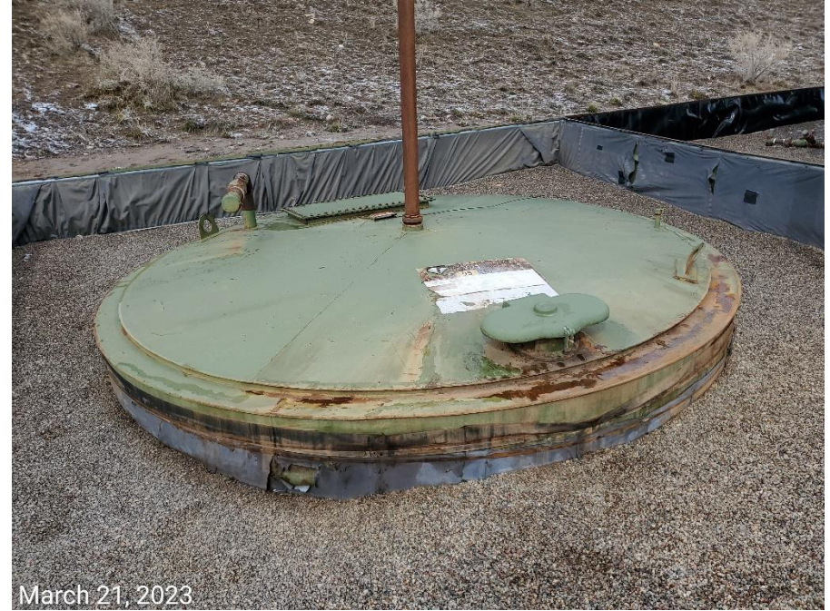
Photo 6: Photos show liner integrity, and tank labeling corrective actions have not yet been addressed.
