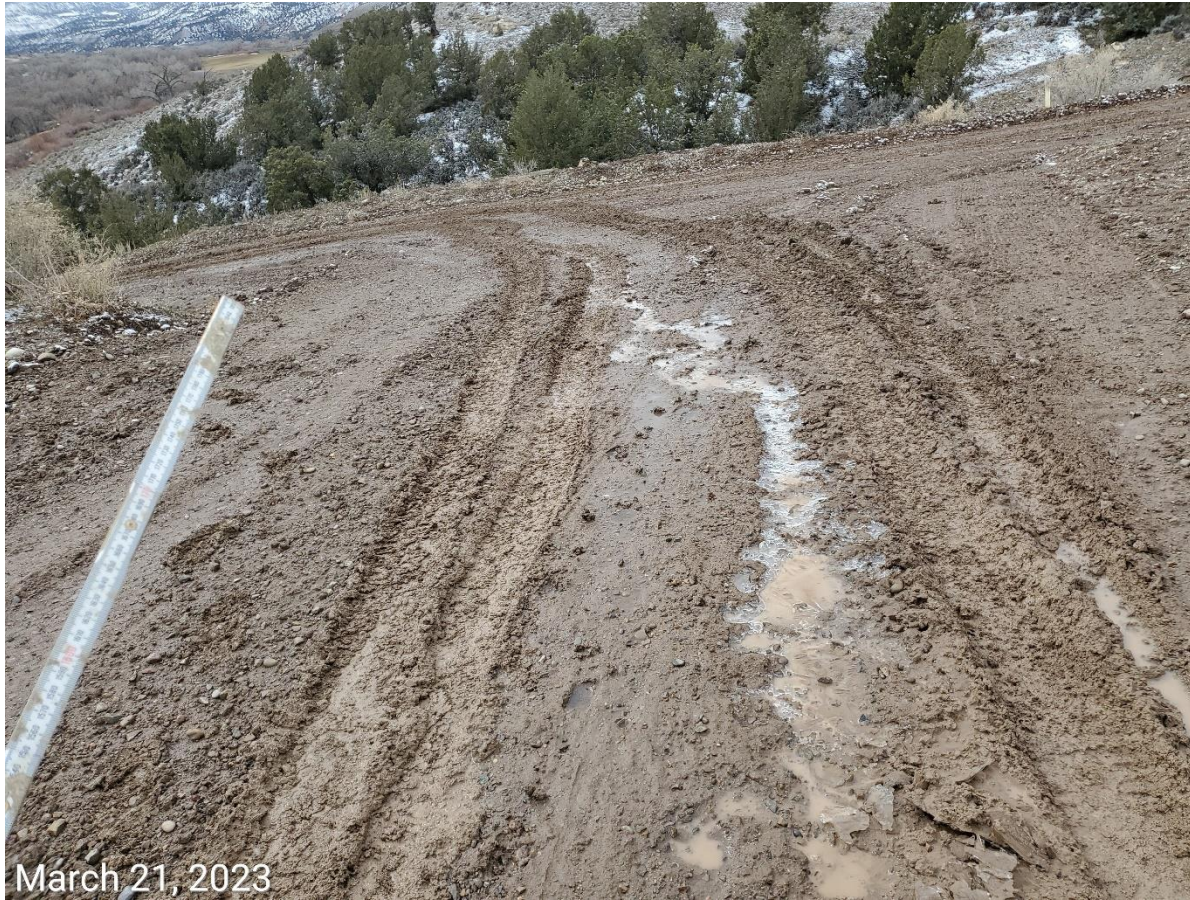
Photo 1: Photos 1-3 taken from Location entrance and access road. Operator appears to have graded road/pad since previous inspection. Photos examples showing BMPs, including vehicle tracking control measures, remain missing or insufficient to minimize erosion, degradation, tracking and sediment transport during wet conditions. Regrading alone is inadequate to address tracking and stabilization issues.
