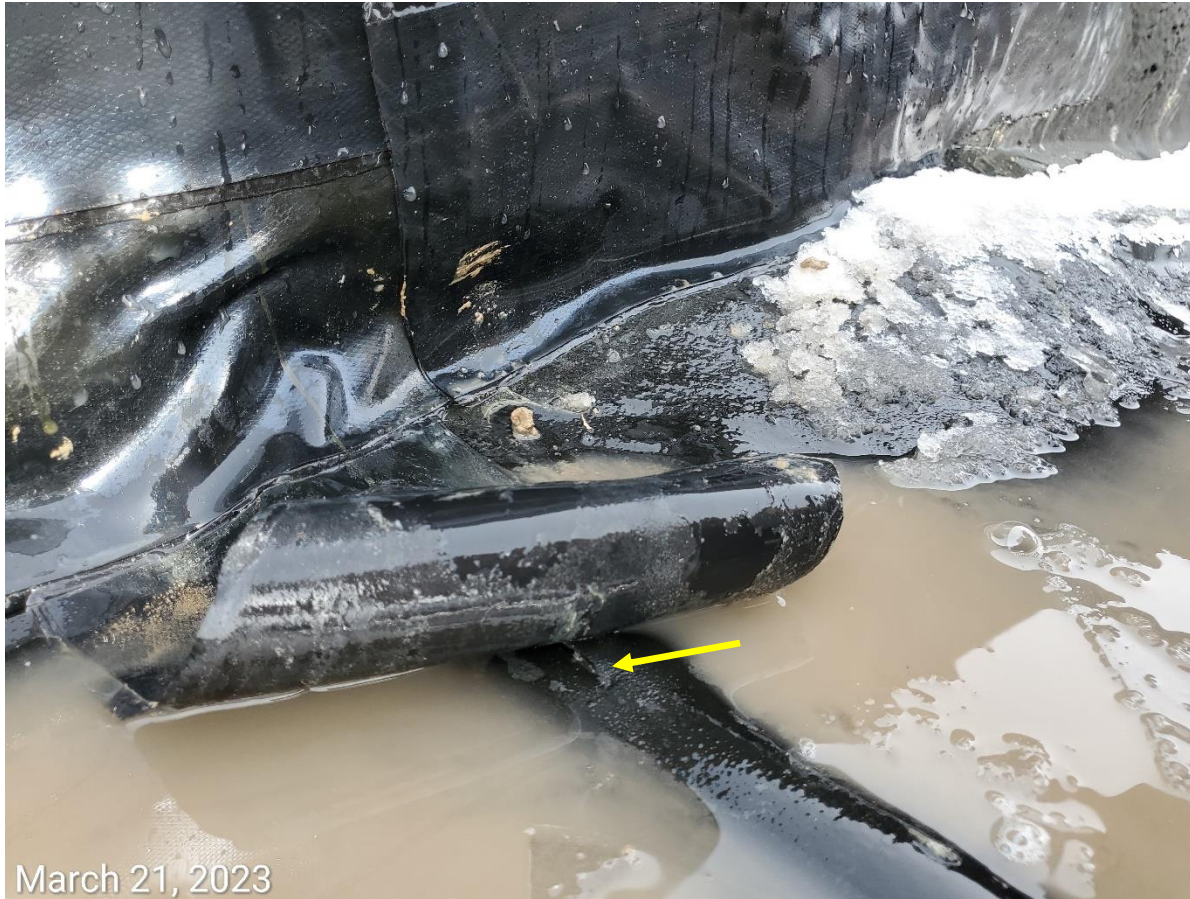
Photo 3: Photo shows repair work at secondary containment liner is inadequate.
