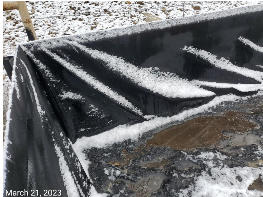
Photo 7: Photo show secondary containment at the tank battery; liner appears to have been repaired.
