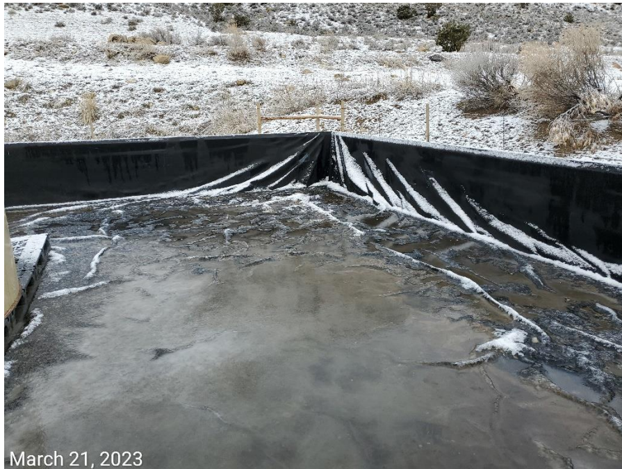
Photo 7: Photo show secondary containment at the tank battery; liner appears to have been repaired.
