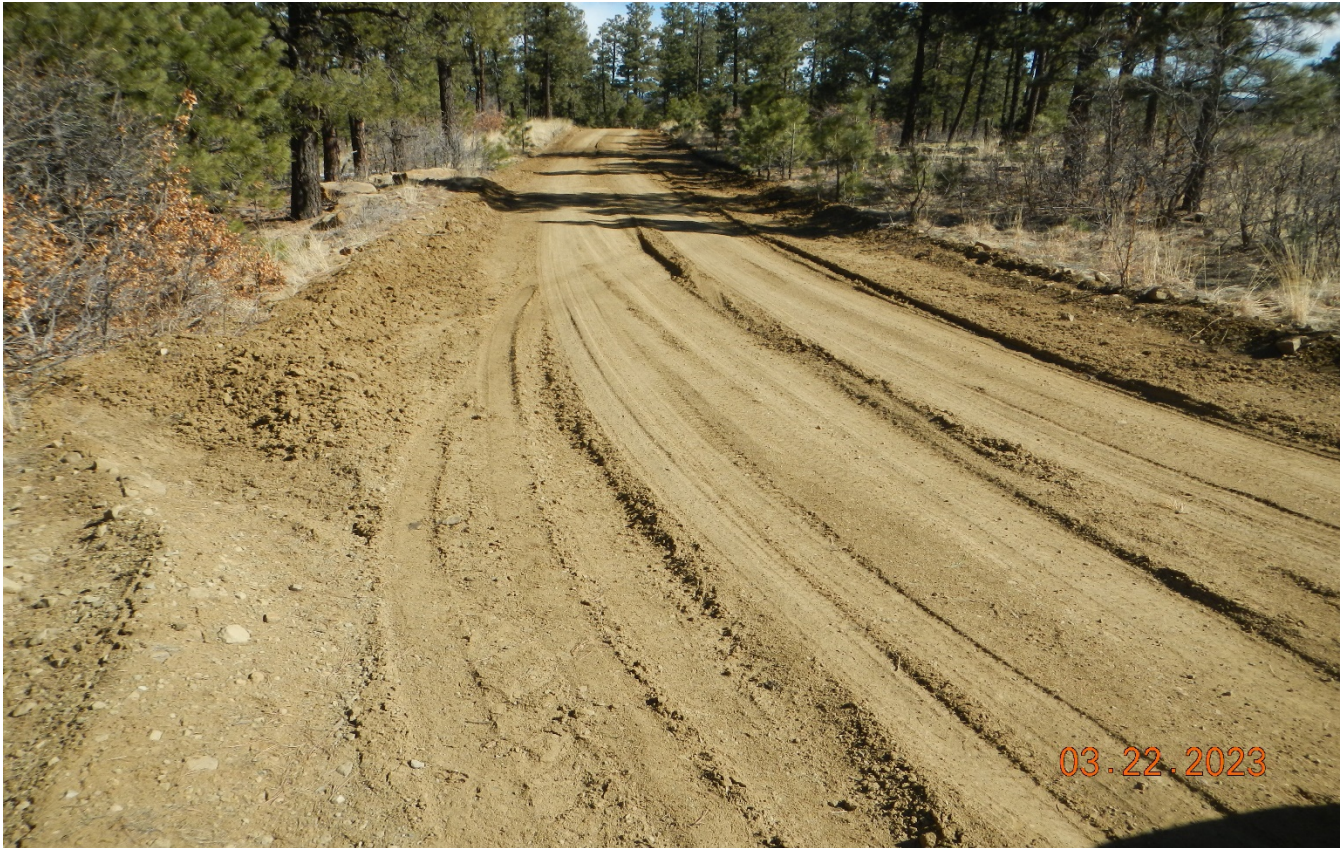
Photo 1. Facing northeast toward the access. Areas of the road are rutted and need to be stabilized.
