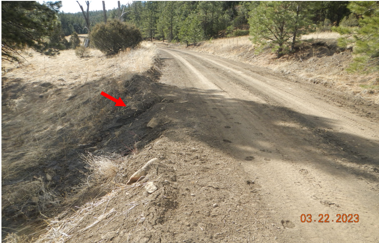
Photo 2. There is an erosion gully along the road that needs to be repaired and stabilized. It appears grading operations has partially filled in this gully however it still needs to be stabilized. Previous corrective action was not completed.
