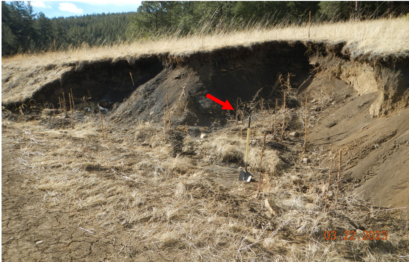
Photo 4. The side of the road is eroded and not stabilized. Erosion head cutting is continuing to occur further back into the slope. This area needs to be repaired and stabilized. Previous corrective action not completed. Red arrow points to 4.5 ft. shovel. Lat/Long:36.99952,-104.83425.
