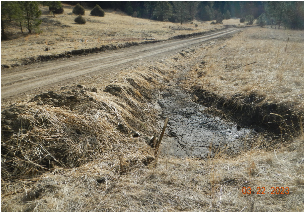
Photo 1. This culvert inlet was cleaned out by the Operator however, the culvert is full of sediment and the inlet has filled back in with sediment. Previous corrective action was not completed. Lat/Long:37.00581,-104.83861.
