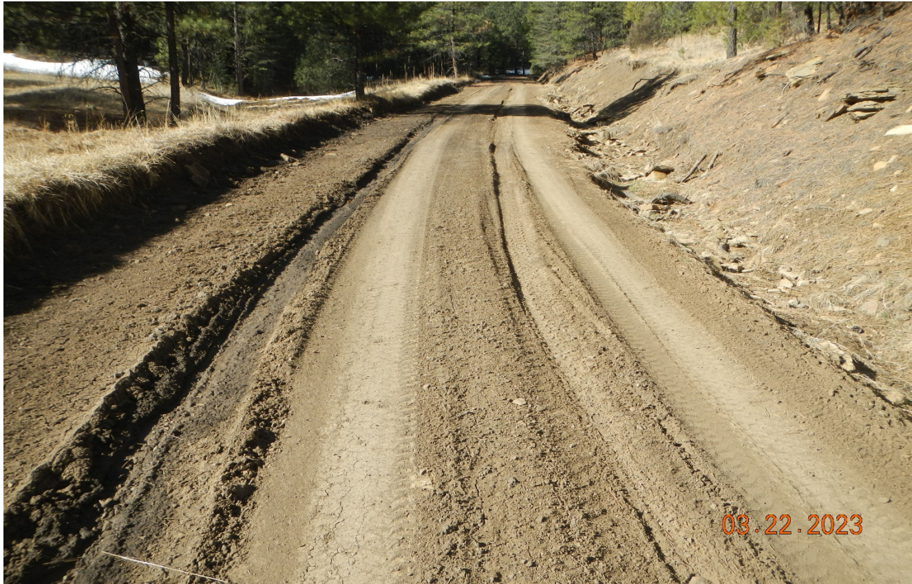
Photo 5. Further along the road near the Colorado line. The roadside and road is eroded and needs to be repaired and stabilized. Previous corrective action not completed.
