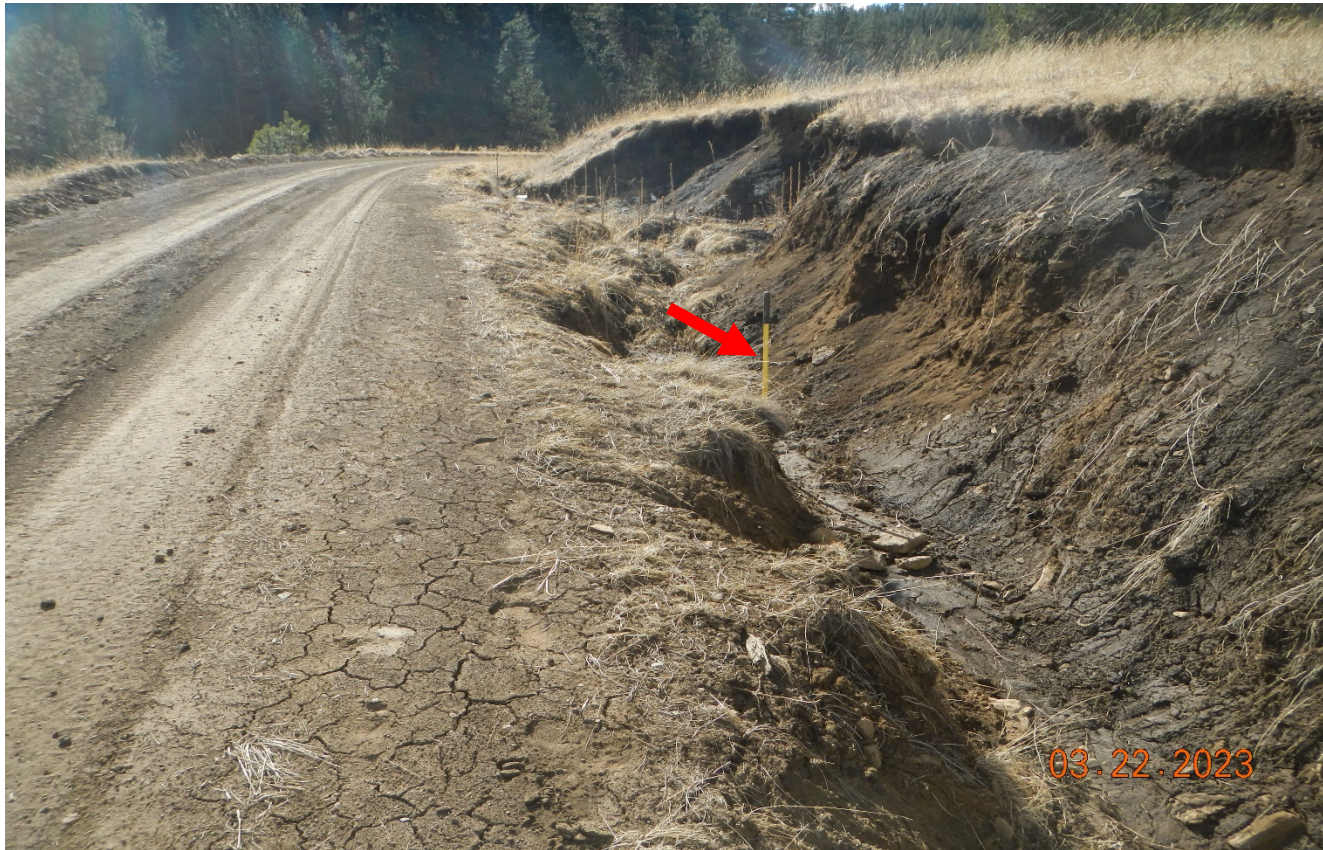
Photo 3. The side of the road is eroded and not stabilized. Erosion head cutting is continuing to occur further back into the slope. This area needs to be repaired and stabilized. Previous corrective action not completed. Red arrow points to 4.5 ft. shovel. Lat/Long:36.99952,-104.83425.
