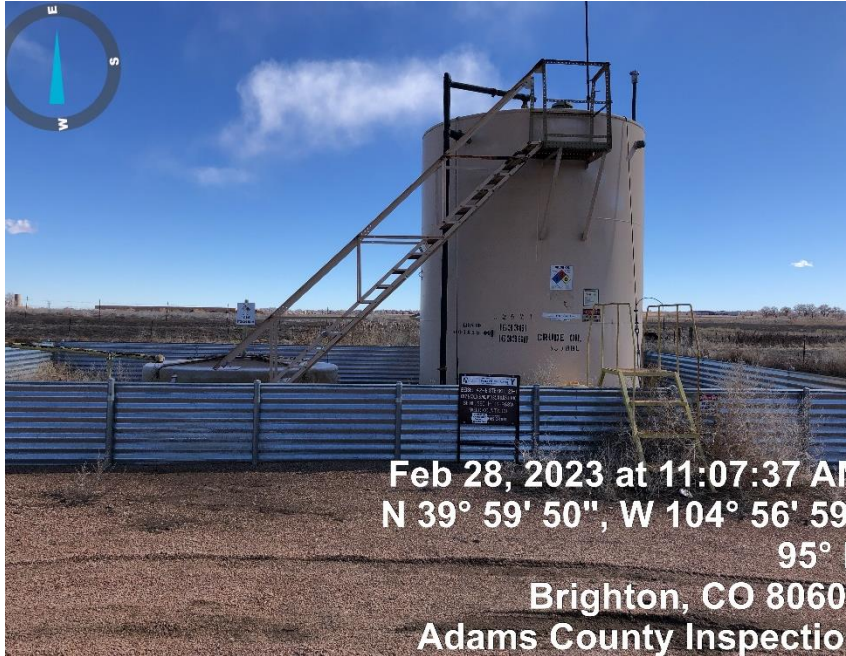
Photo#1 Production Tank and Produced Water Tank
