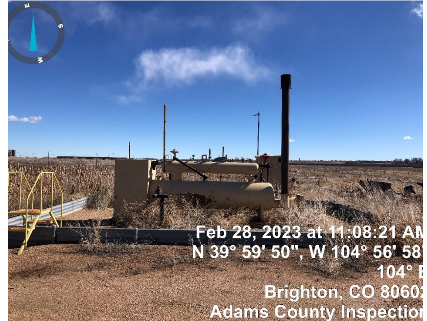
Photo#2 Separator/Gas Meter
