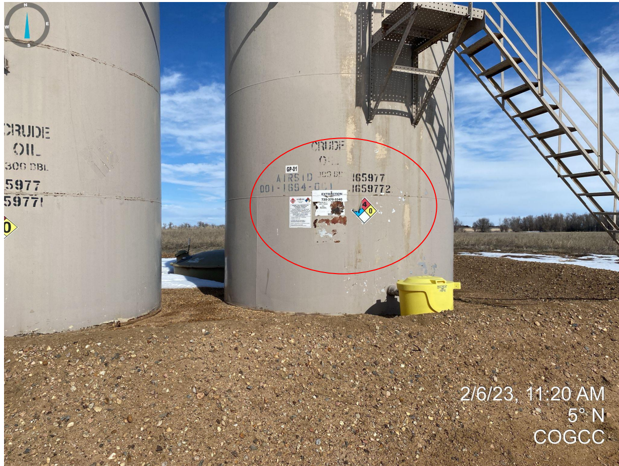
Photo 4. Facing north at the tank battery; photo illustrates that the NFPA placards and other labels on the tank are peeling, cracked, and not legible.
