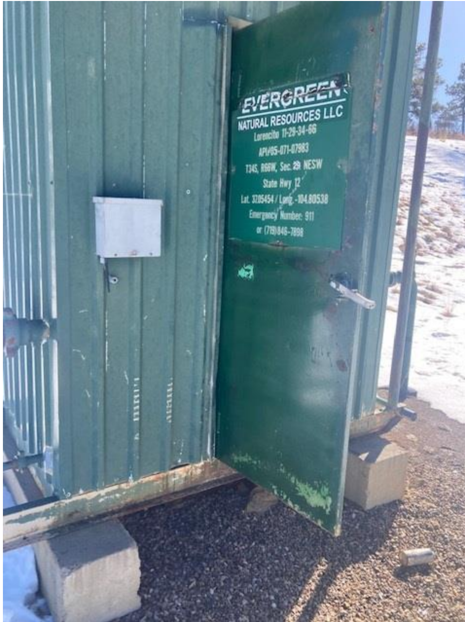
Fixed Hinge on door Secured and fastened all valves, pipes, and fittings to ensure good mechanical condition, inspected at regular intervals and maintained in good mechanical condition per Rule 608.e.
