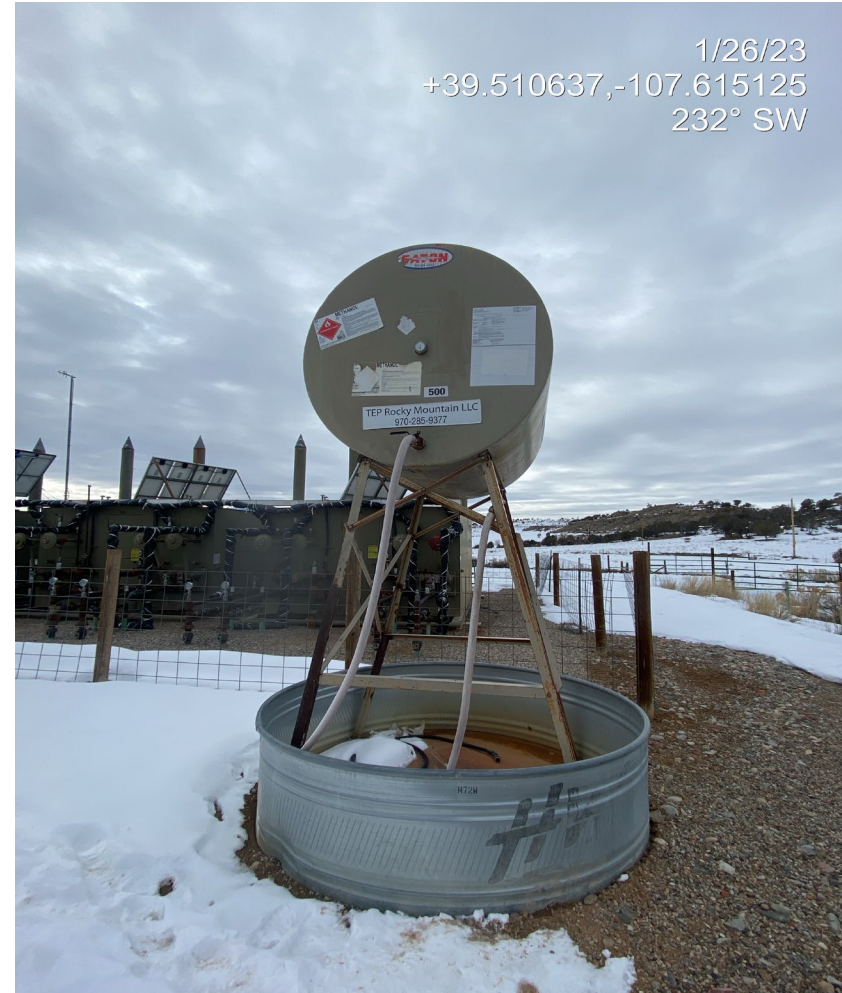
Photo 2. Photos show staining beneath well API # 045-08454 (left) and wildlife protection BMPs missing on a secondary containment stock tank (right).
