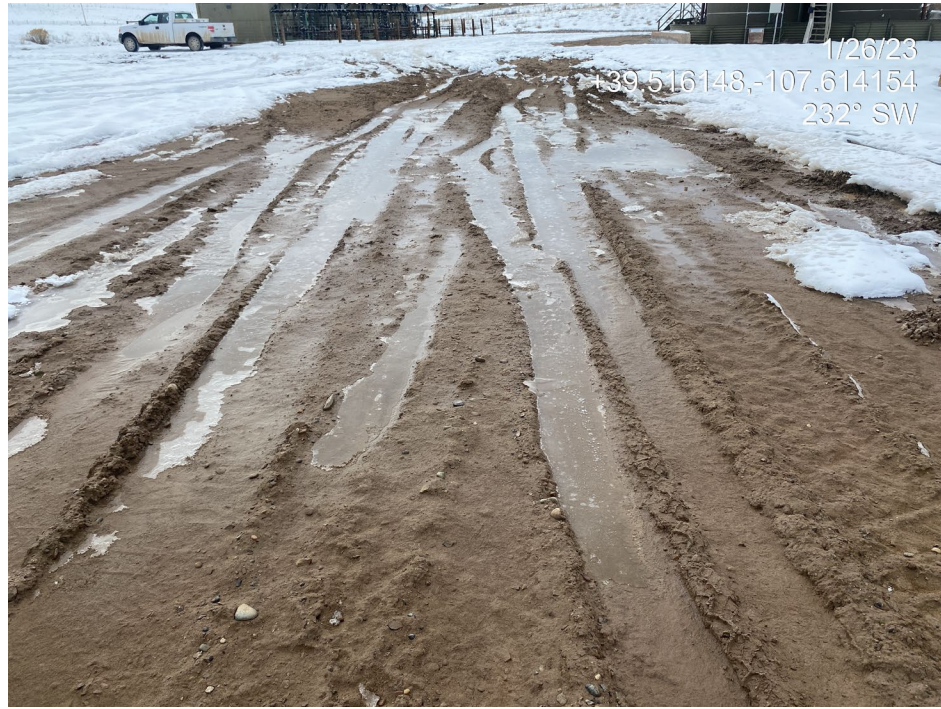
Photo 3. Photos show degradation to the pad surface and lack of stabilization BMPs and tracking controls.
