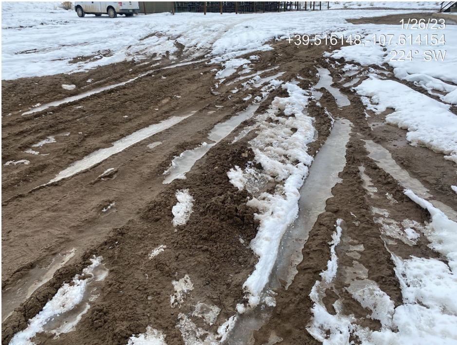
Photo 4. Photos show degradation to the pad surface and lack of stabilization BMPs and tracking controls.
