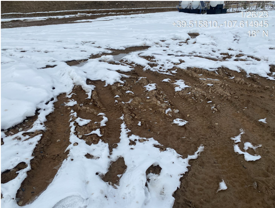
Photo 3. Photos show degradation to the pad surface and lack of stabilization BMPs and tracking controls.
