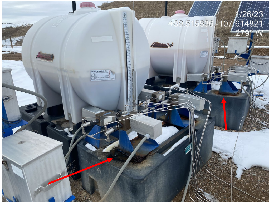
Photo 2. Photos show leaky chemical injection units.
