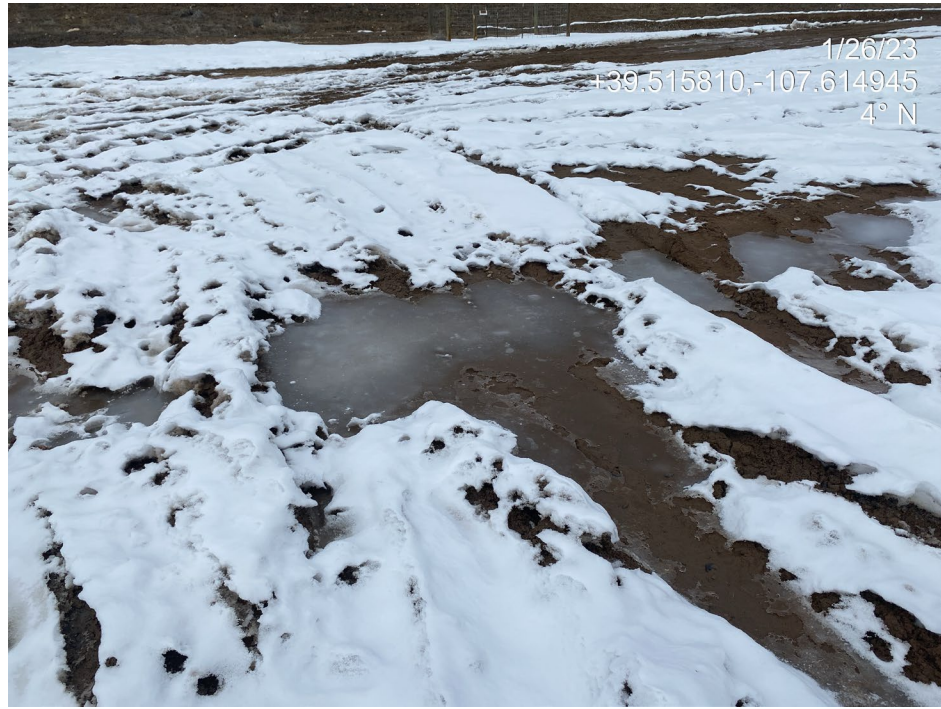
Photo 4. Photos show degradation to the pad surface and lack of stabilization BMPs and tracking controls.
