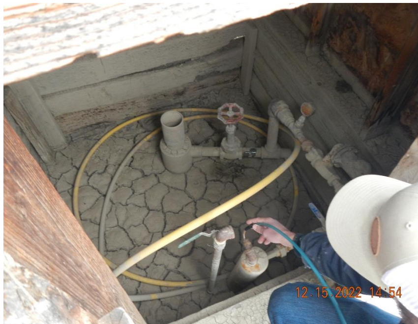
Cottonwood Consulting attempting to detect leaks from the Bert Eaton (OWP) #1.
