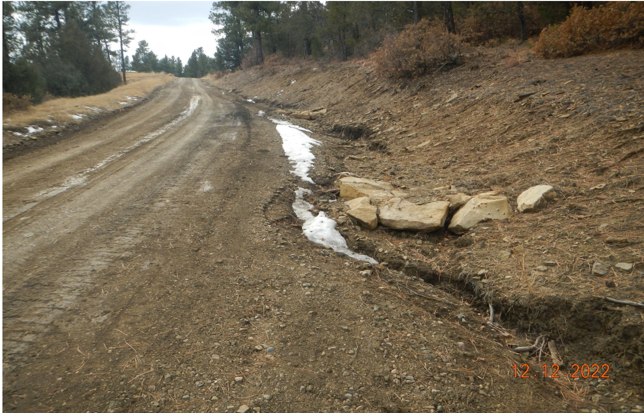
Photo 4. There was repairs made since previous inspection however erosion is occurring around the rock check dams. BMP maintenance is needed and additional BMP's should be installed.
