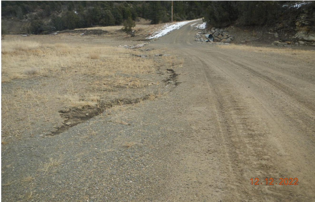
Photo 1. Facing east toward the access road stream crossing. There is erosion beginning to occur in this area and needs to be repaired.
