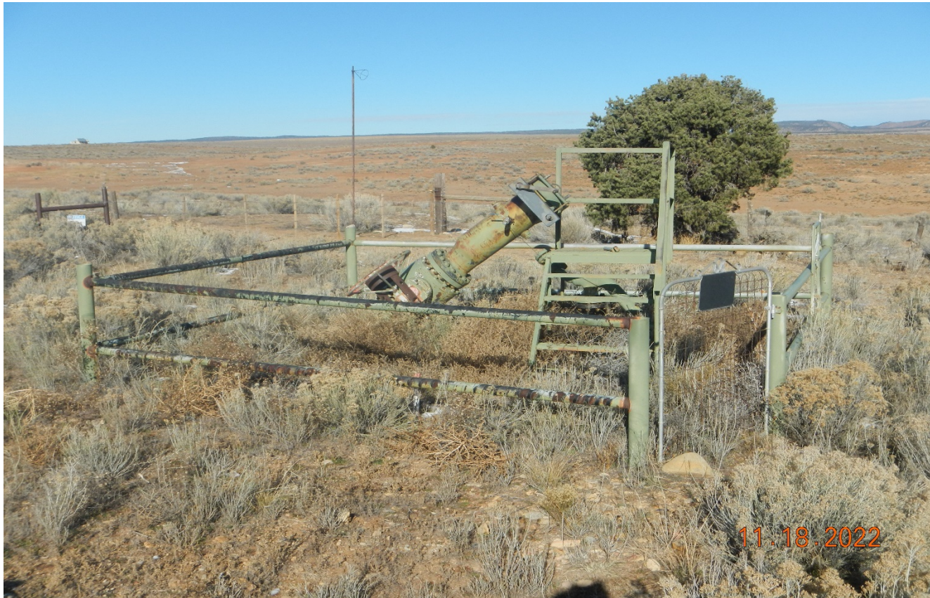
Photo 1. There is a pig launcher that remains approximately 1900' NW of the location. All equipment needs to be removed. Lat/Long:37.15495,-108.17333.
