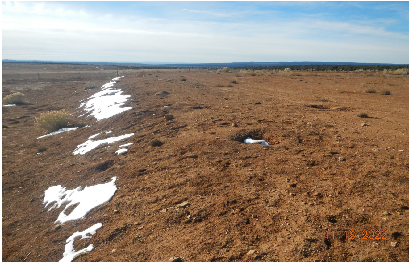
Photo 5. Facing south toward the fill slope at the east side of the location. The fill slope material is approximately 6' from original grade.
