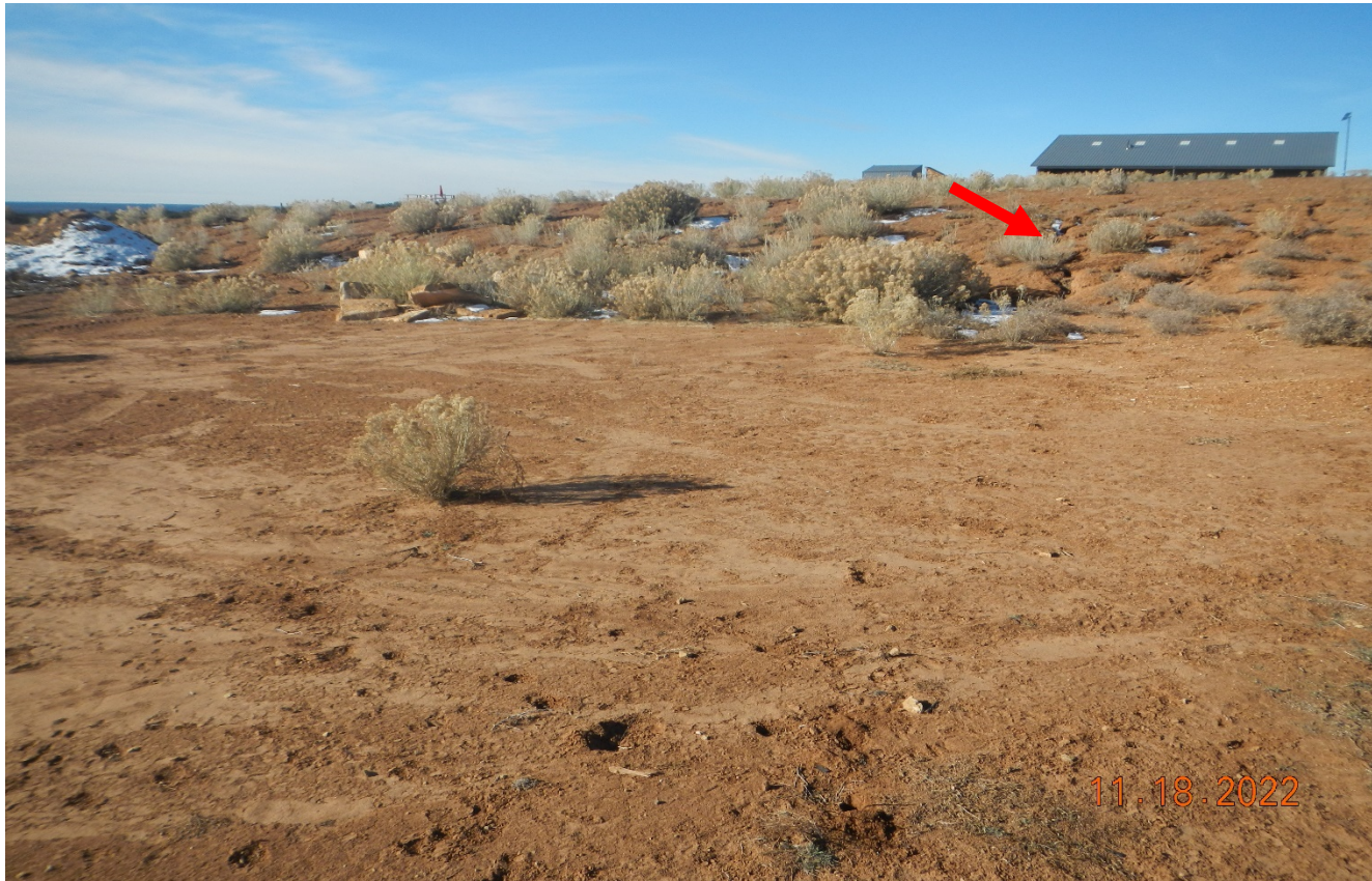
Photo 4. Facing west toward the cut slope which is approximately 6-8 ft. from original grade. There are signs of erosion along the cut slope shown at red arrow.
