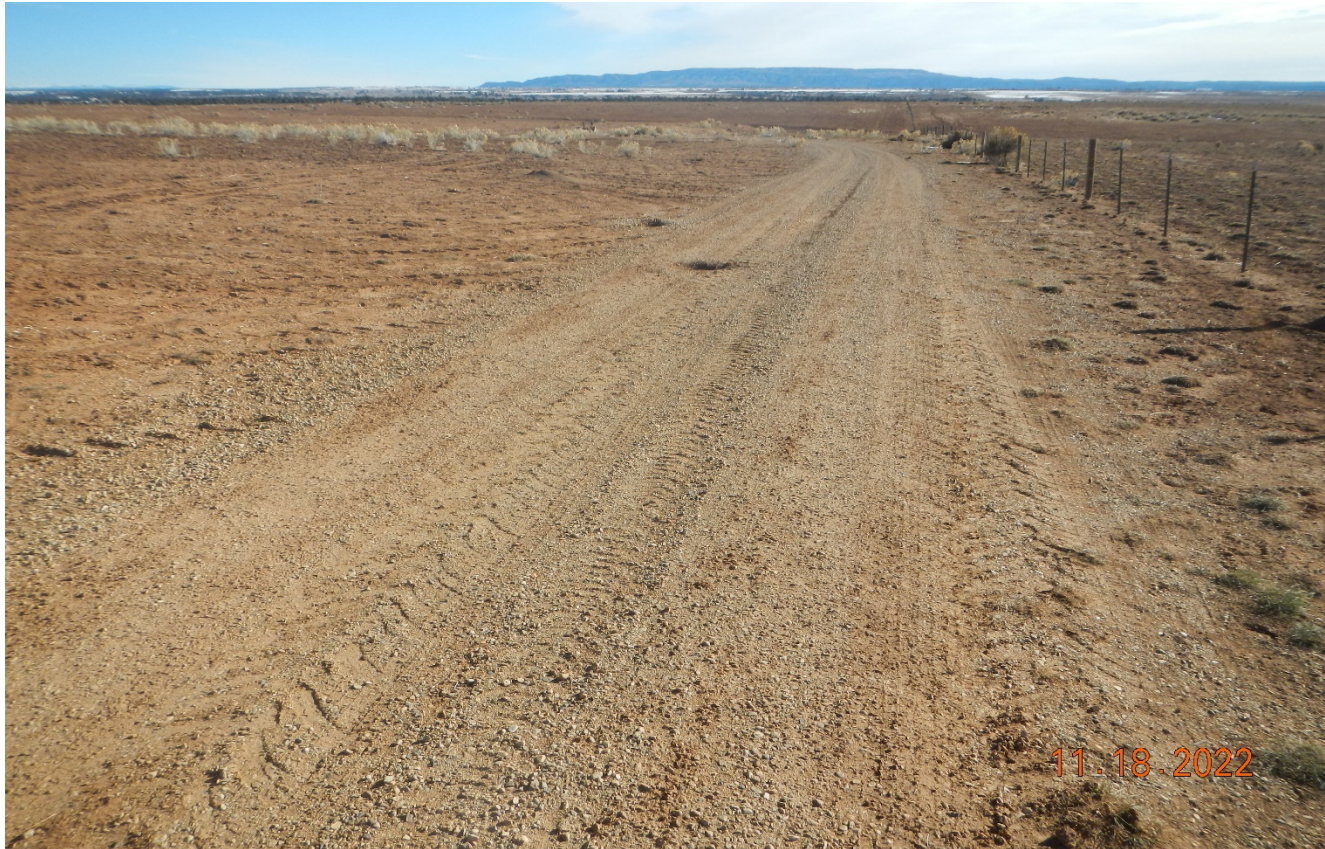
Photo 2. Facing east along the access road which has not been reclaimed and gravel remains.
