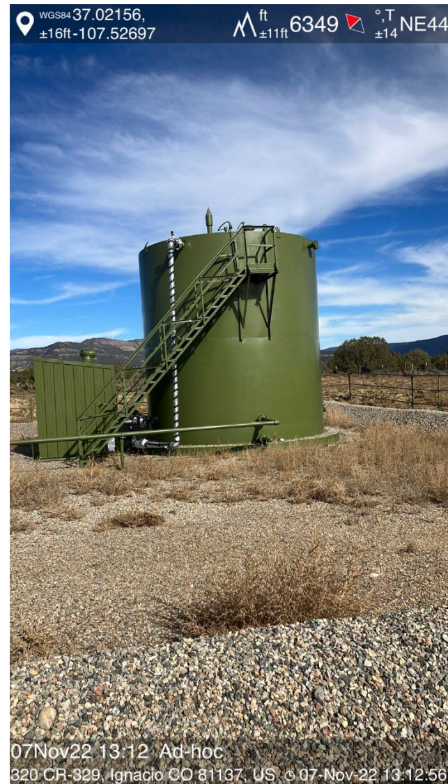
IMG 06 Produced water tank
