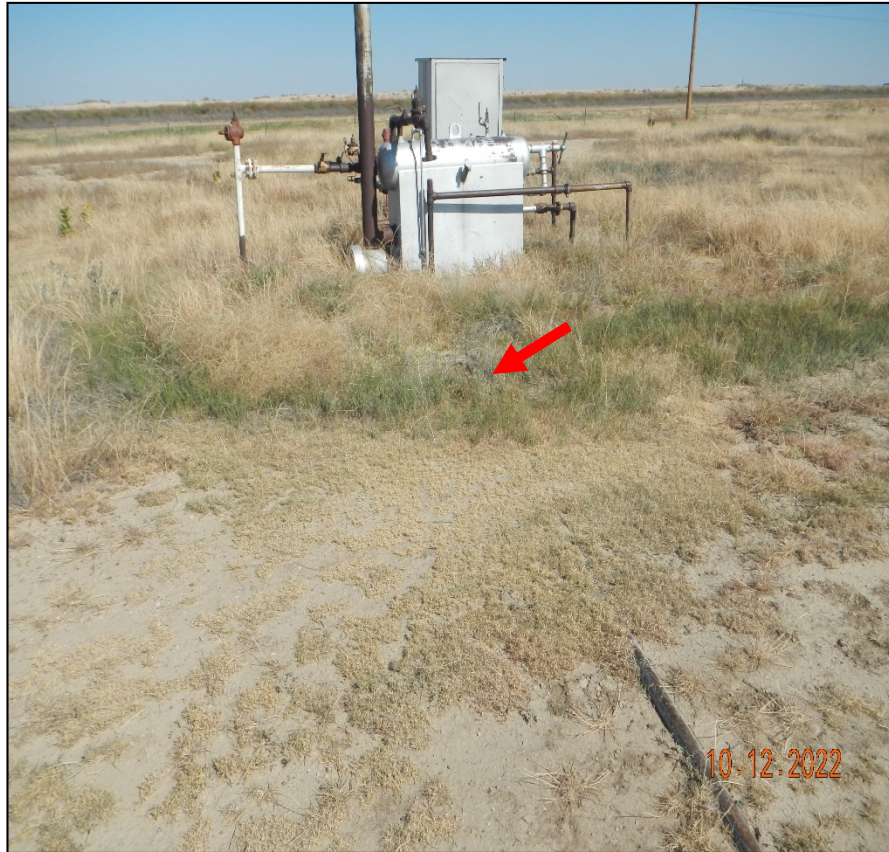
Photo 7. This flowline had previously leaked at red arrow.
