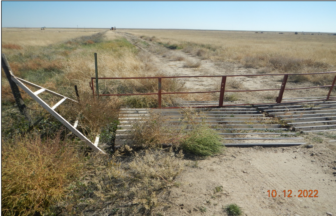
Photo 1. Facing east at the beginning of the access road. The cattleguard is filled in with sediment and needs to be cleaned out and maintained. There is a heavy red panel wired to prevent livestock from crossing cattleguard which makes it difficult to access.
