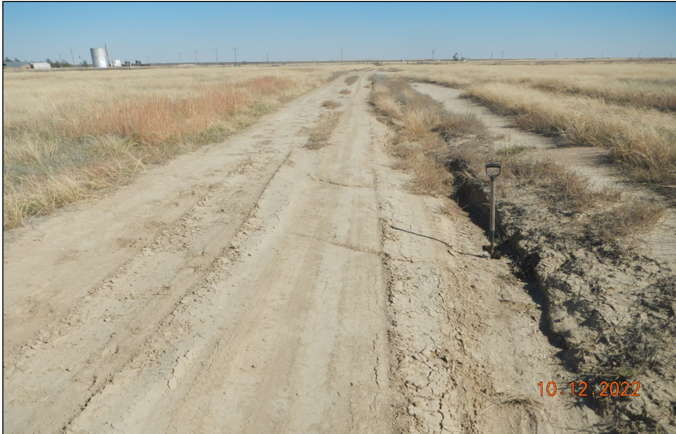
Photo 2. Facing northeast along the access road. There is erosion along the road that needs to be repaired. Vehicles are avoiding this area causing widening of the road.
