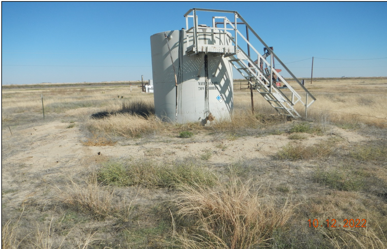
Photo 3. Facing toward the tank battery. The area inside the berm needs to be kept free of vegetation. The fence around the tank needs to be repaired to prevent livestock entry. The berm around the tank needs to be rebuilt to contain a spill.
