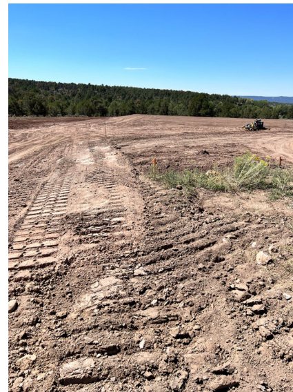
Wattles reinstalled. Erosion channeling addressed when road to Tiffany 5 pad installed. Date completed 9/01/2022
