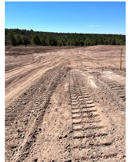
Wattles reinstalled. Erosion channeling addressed when road to Tiffany 5 pad installed. Date completed 9/01/2022
