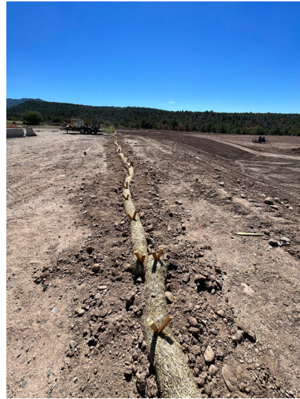
Wattles reinstalled. Erosion channeling addressed when road to Tiffany 5 pad installed. Date completed 9/01/2022
