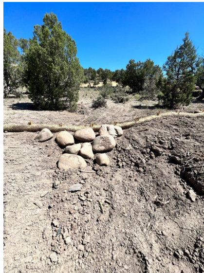
Wattles reinstalled. Erosion channeling addressed when road to Tiffany 5 pad installed. Date completed 9/01/2022
