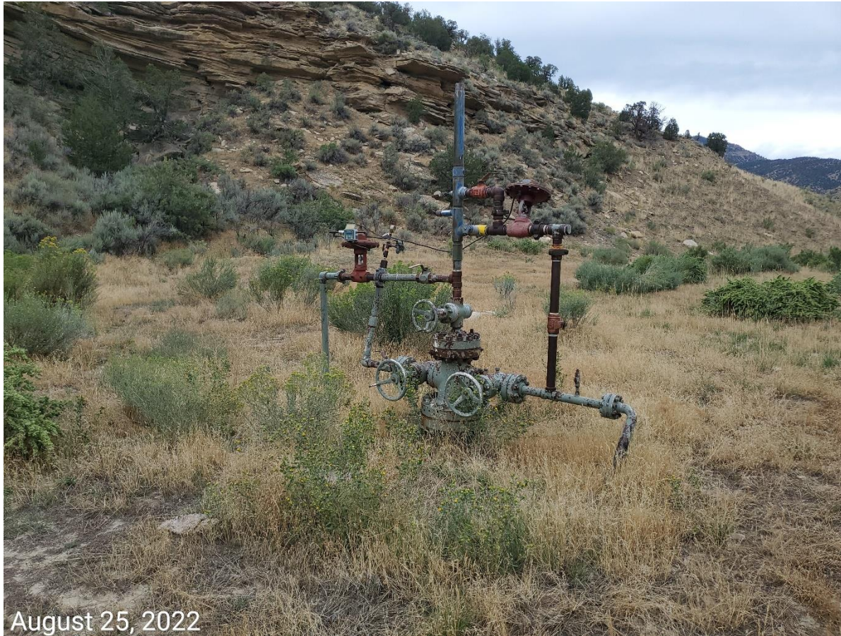
Photo 1: Well head- signage missing
