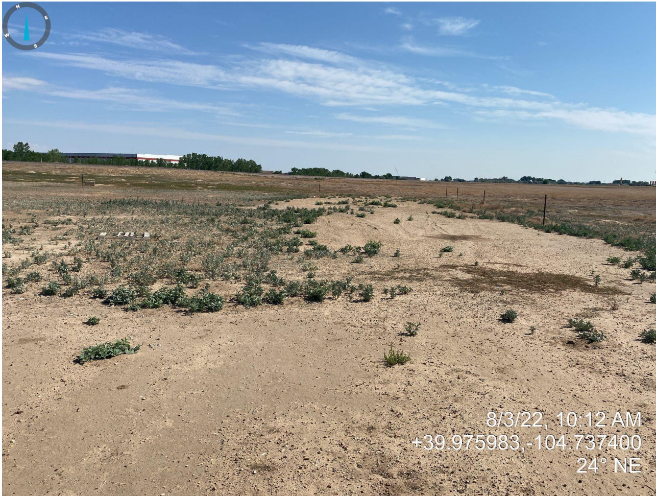
Photo 2. Photo taken from southern portion of location, facing northeast. Location has not been reclaimed and revegetated resulting in bare soil. Debris and gravel/road base remain on site.
