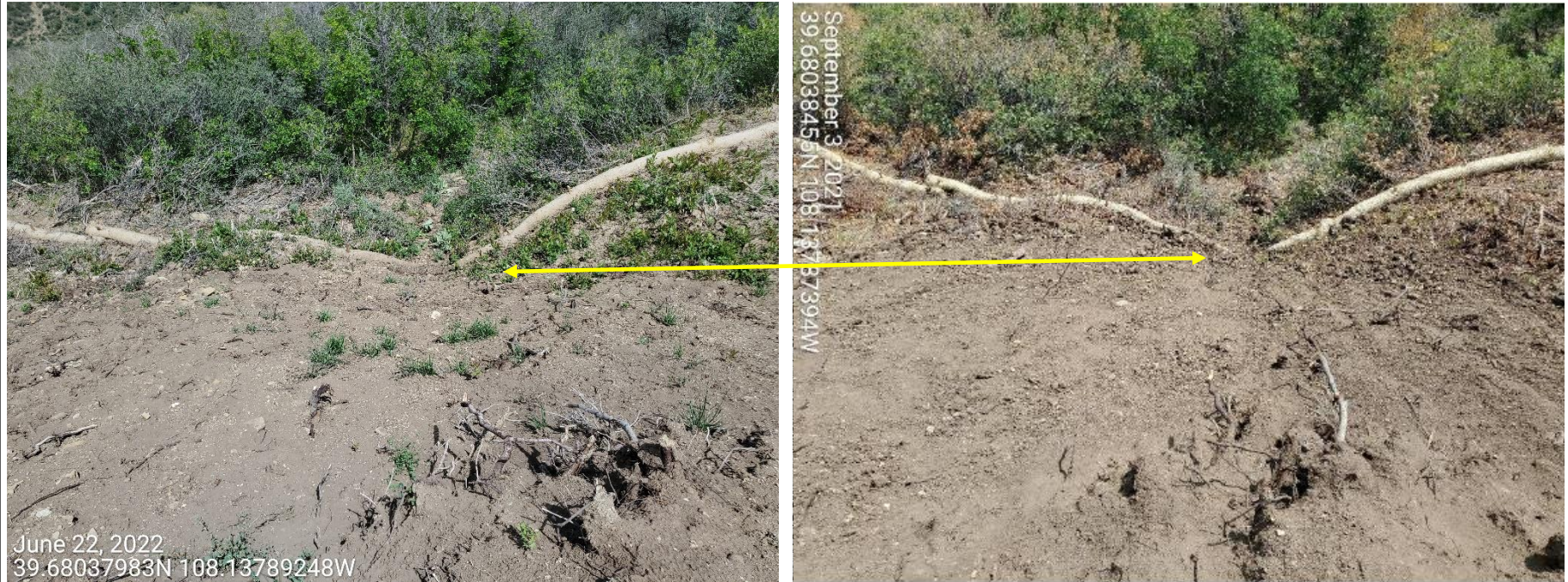
Photo 4: Photos taken from the perimeter of the Location. Photo left shows BMPs to minimize erosion , degradation and sediment transport at topsoil stockpiles have not been maintained; off-site sediment transport observed (arrows). Photo left dated 6/22/2022, photos right dated 9/3/2021- sediment transport observed in previous inspection occurring in the same spot.
