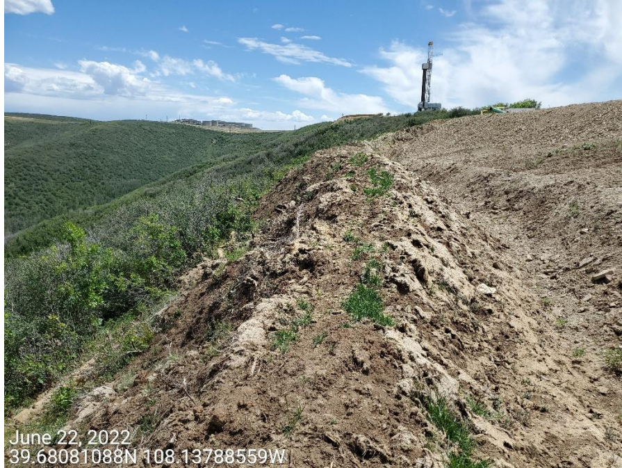
Photo 3: Photos taken from the perimeter of the Location. Photos examples showing that topsoil remains in use at the base of the fill slopes/subsoils of the Location as a berm and sediment trap/pond to manage stormwater. BMPs to minimize erosion and degradation at topsoil stockpiles have not been maintained.
