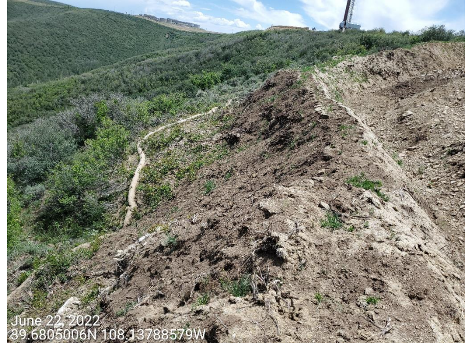
Photo 3: Photos taken from the perimeter of the Location. Photos examples showing that topsoil remains in use at the base of the fill slopes/subsoils of the Location as a berm and sediment trap/pond to manage stormwater. BMPs to minimize erosion and degradation at topsoil stockpiles have not been maintained.
