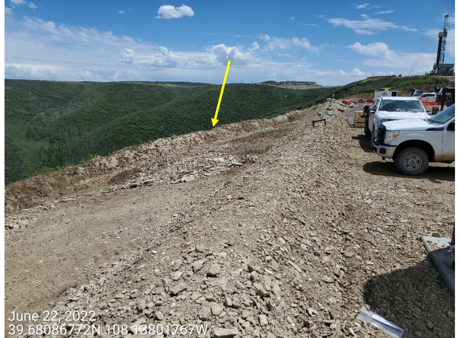
Photo 2: Photos taken from the perimeter of the Location. Photos examples showing that topsoil remains in use at the base of the fill slopes/subsoils of the Location as a berm and sediment trap/pond to manage stormwater. BMPs to minimize erosion and degradation at topsoil stockpiles have not been maintained.
