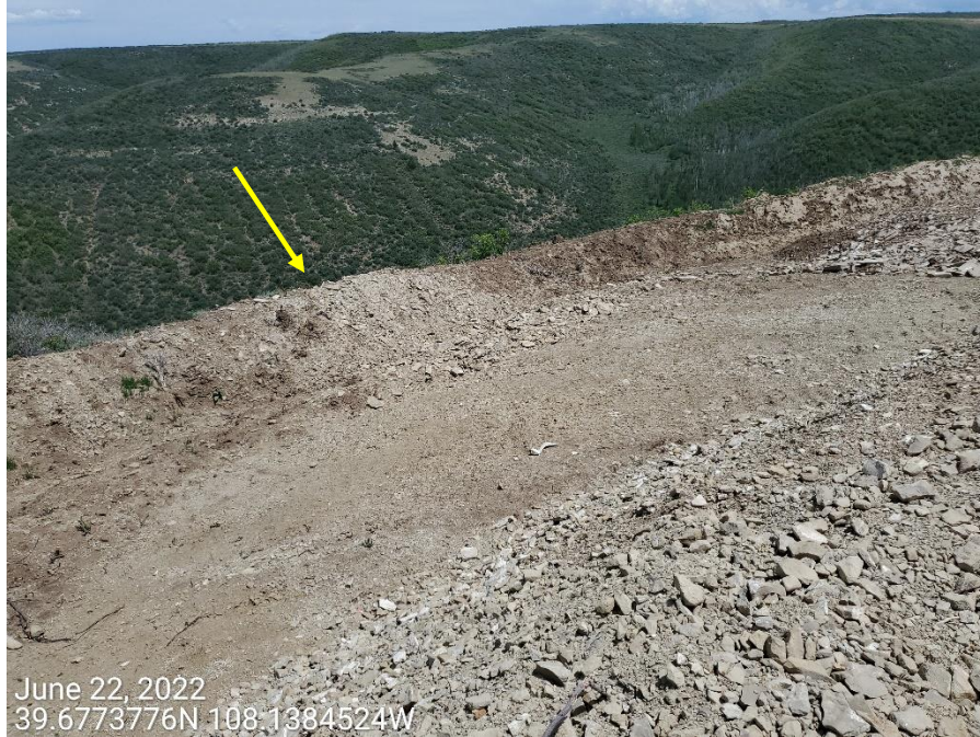
Photo 2: Photos taken from the perimeter of the Location. Photos examples showing that topsoil remains in use at the base of the fill slopes/subsoils of the Location as a berm and sediment trap/pond to manage stormwater. BMPs to minimize erosion and degradation at topsoil stockpiles have not been maintained.
