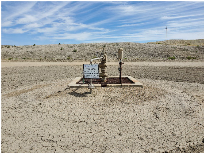
Injection wellhead.
